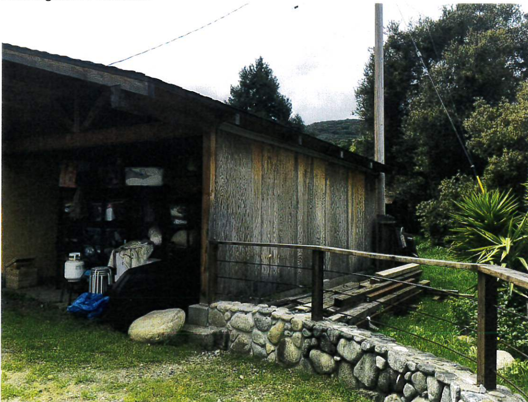
Shed Rear Elevation
