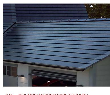
7.14 - TESLA "SOLAR ROOF" ROOF TILES WITH INTEGRATED PV PANELS
