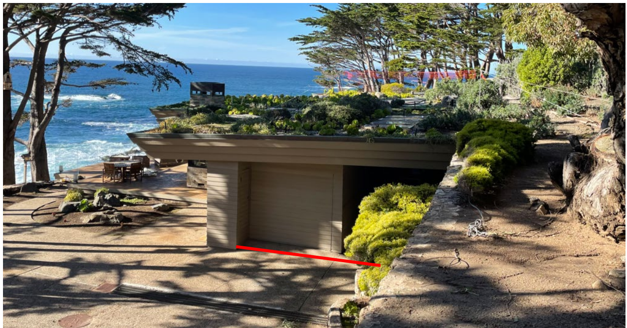
Figure 3: Photo of existing home. Addition will follow line denoted in red, and height addition flagged in orange.
