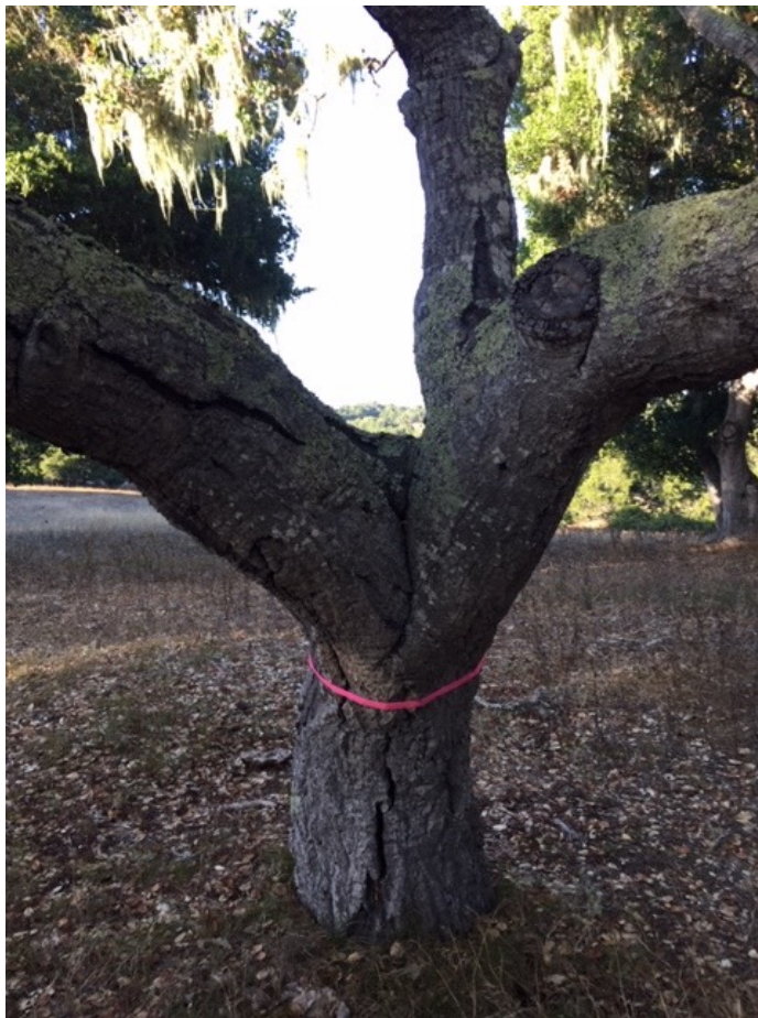
Figure 23. Closer view of Tree#36 that is proposed for removal.
