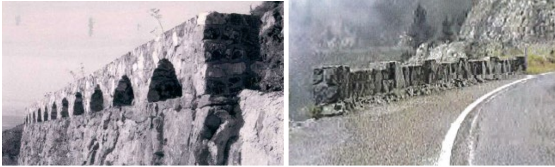
Figure 2: An arcade-style masonry parapet and battlement parapet
