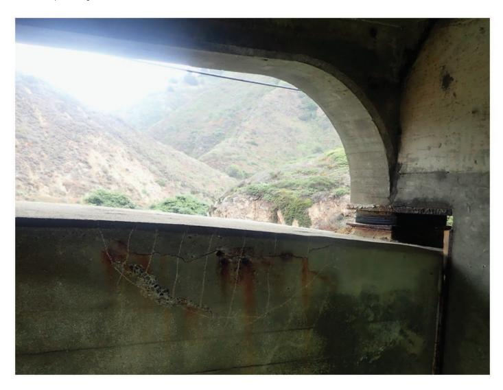
Photo No. 5 Delamination at the left face of the right arch rib adjacent to Spandrel Column 4.
