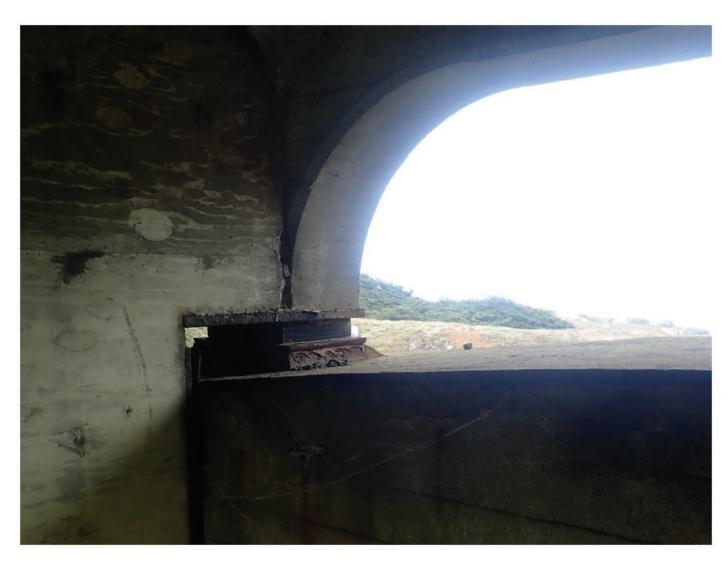
Photo No. 6 Delamination at the right face of the left arch rib adjacent to Spandrel Column 4.
