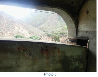
Delamination at the left face of the right arch rib adjacent to Spandrel Column 4.
