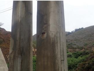
Photo 7 Spall with exposed rebar on the left face of Column 2 at Bent 5.
