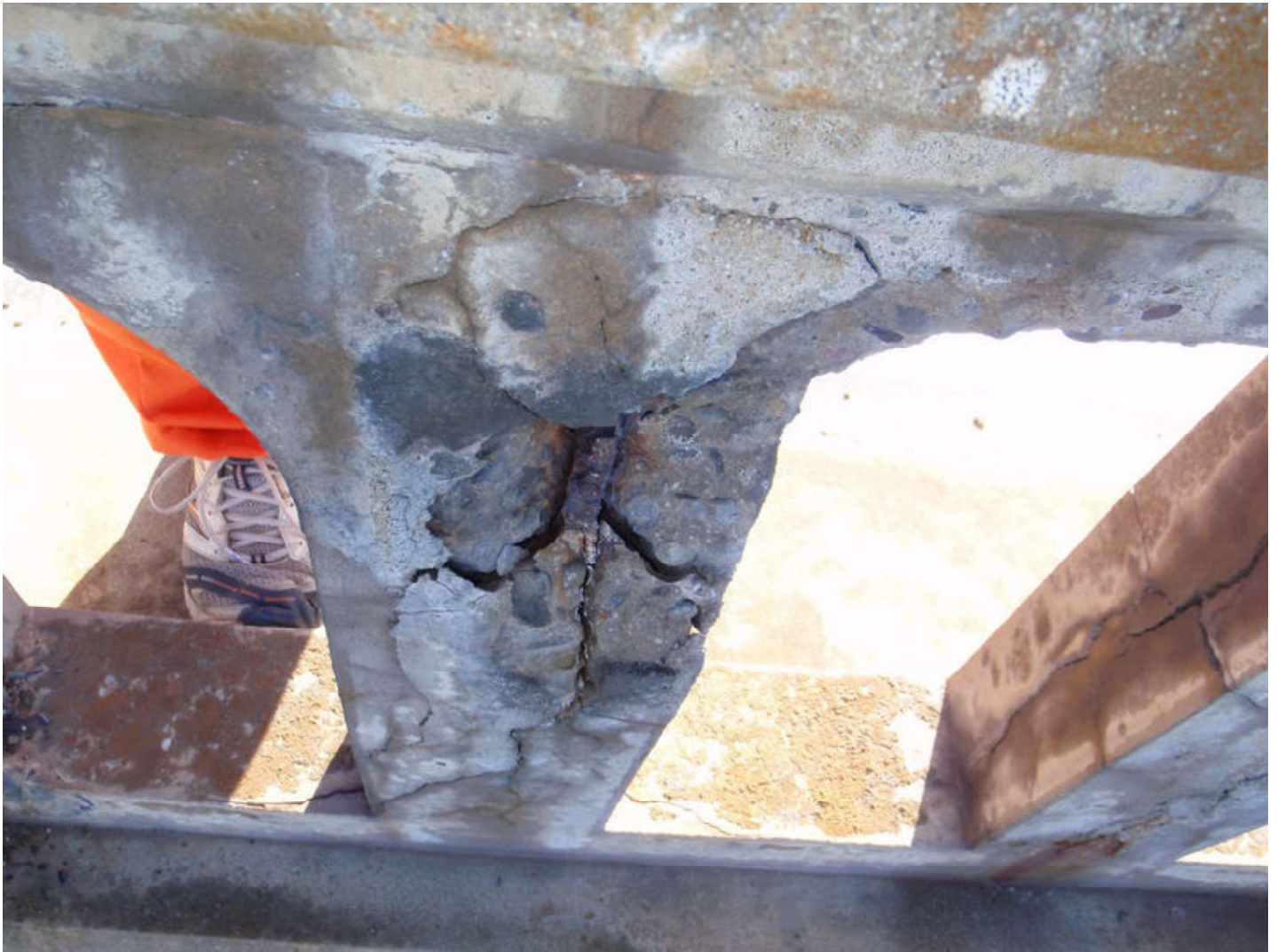
Photo #7 Gross deterioration of bridge railing.
