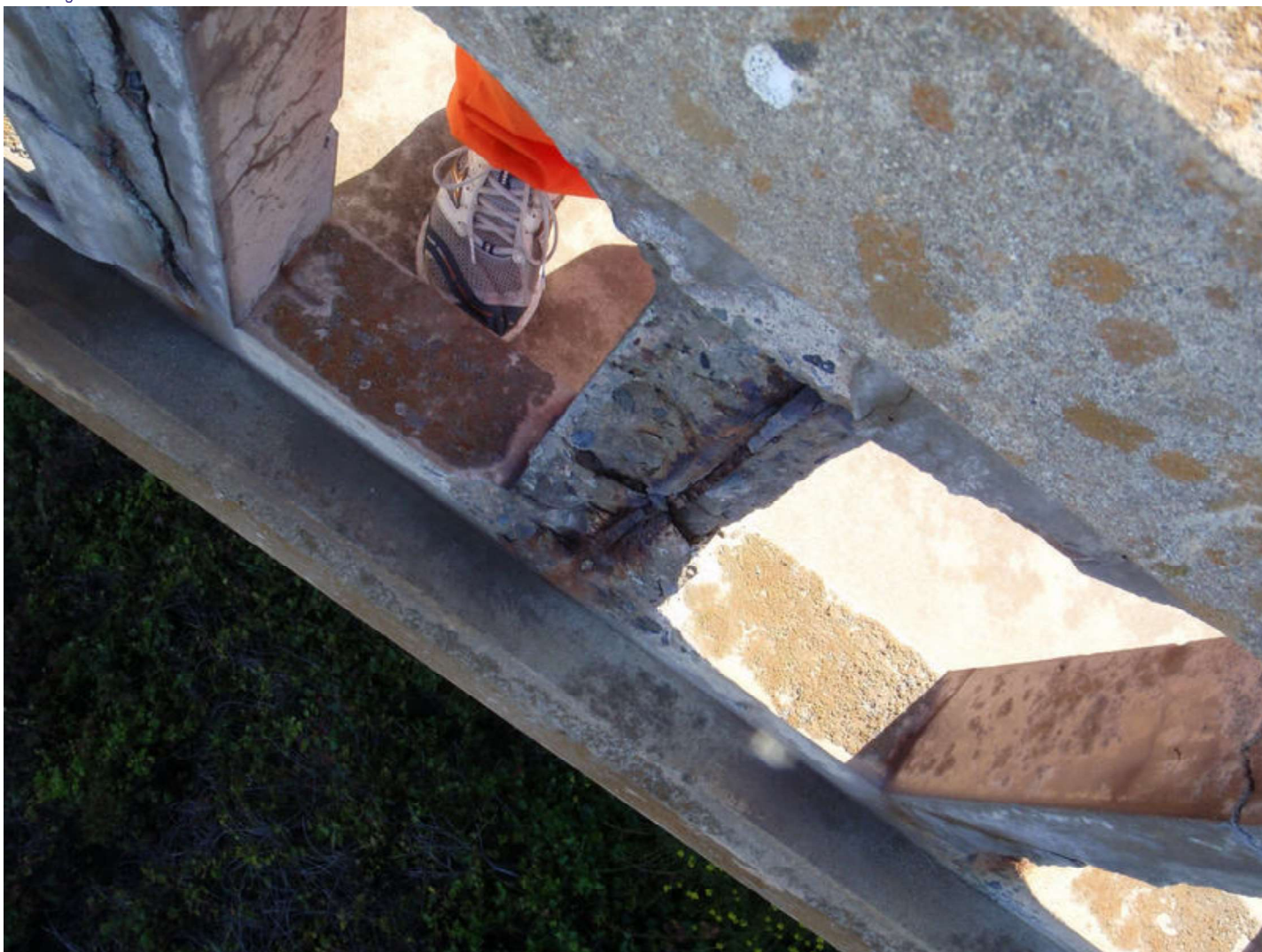
Photo #6 Gross deterioration of bridge railing.
