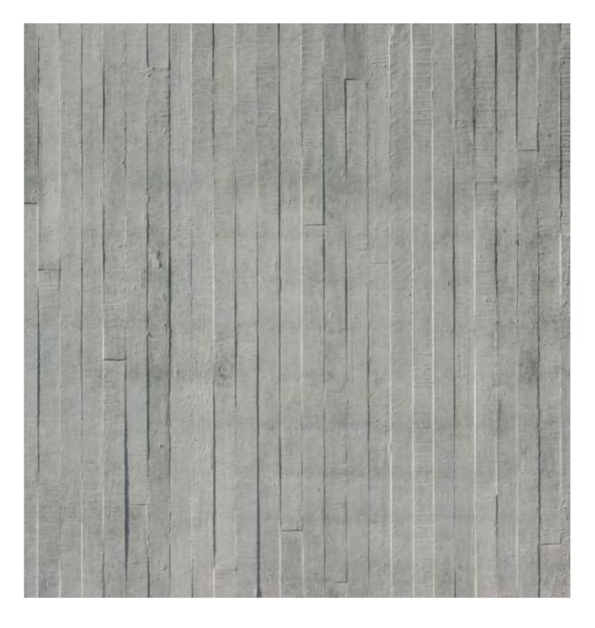
VERTICAL BOARD FORMED CONCRETE -RETAINING WALLS
