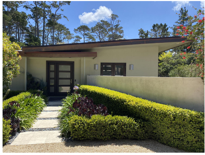
COPPER PAINTED ALUMINUM FASCIA TO MATCH EXISTING
