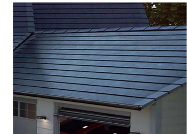
7.14 - TESLA "SOLAR ROOF" ROOF TILES WITH INTEGRATED PV PANELS
