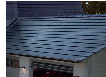
7.14 - TESLA "SOLAR ROOF" ROOF TILES WITH INTEGRATED PV PANELS
