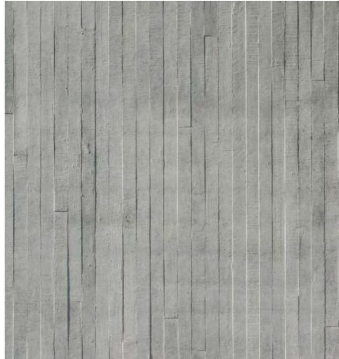
VERTICAL BOARD FORMED CONCRETE - RETAINING WALLS
