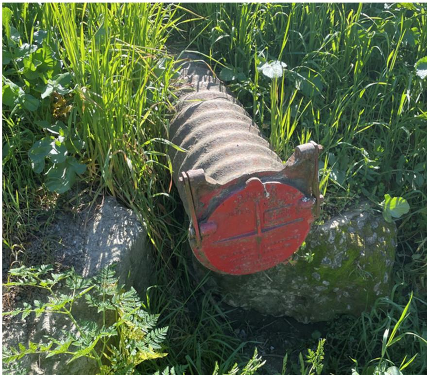
Photo 4. Area B-2 Outfall (12" CMP with flap gate)
