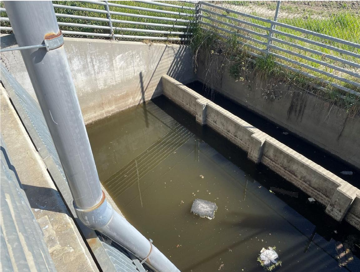
Photo 2. Pump station inlet bay with trash pump suction pipe in foreground
