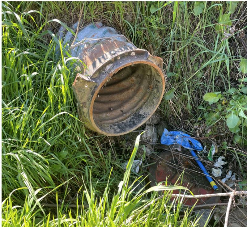
Photo 5. Area B-3 Outfall (15" CMP with broken flap gate)
