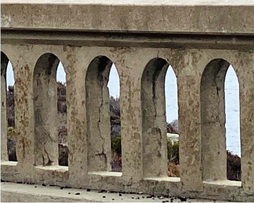
Figure 1-7 Photo of Malpaso Creek Bridge Rail Deterioration
