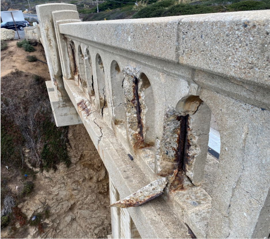
Figure 1-4 Photo of Garrapata Creek Bridge Rail Damage
