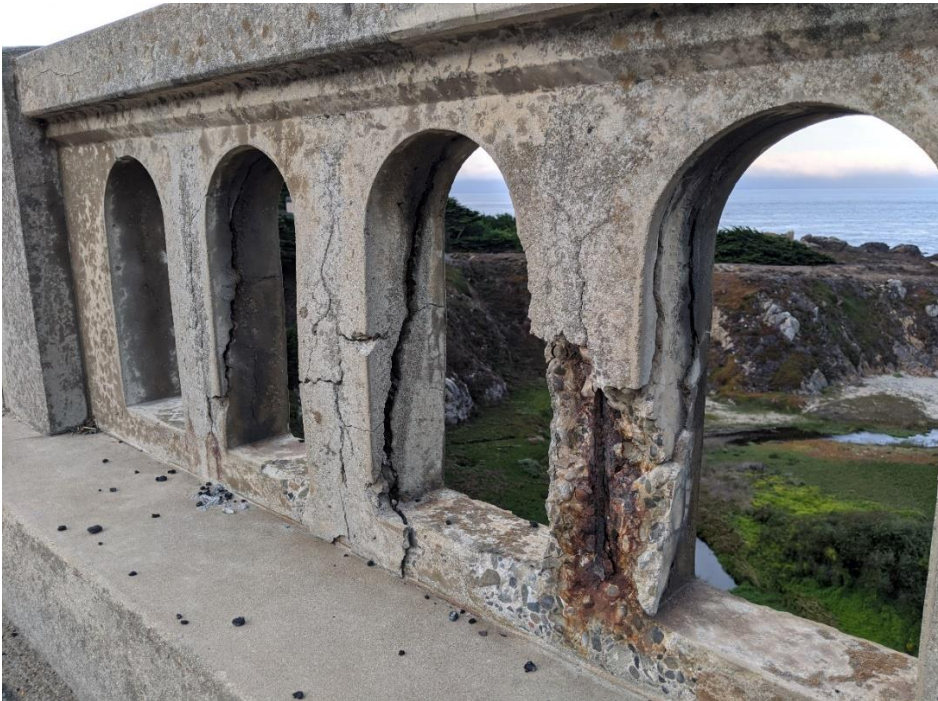
Figure 1-4 Photo of Garrapata Creek Bridge Rail Damage
