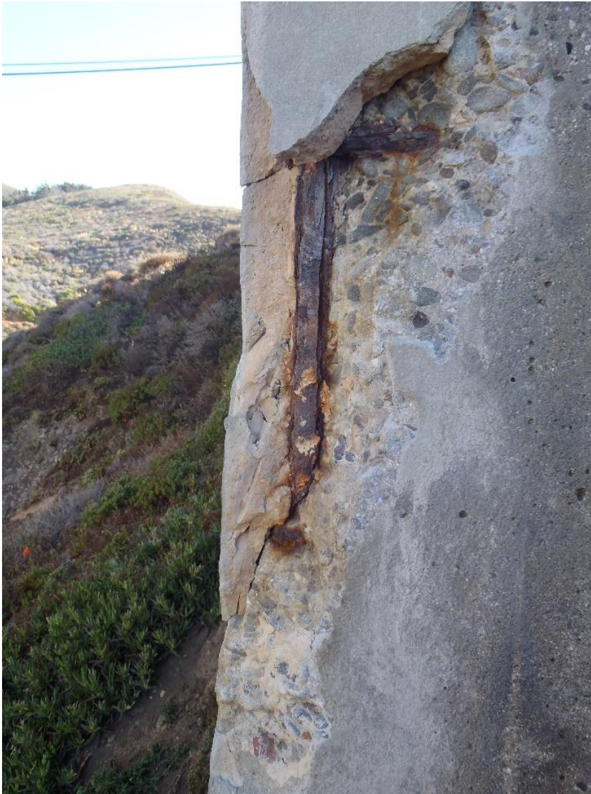
Figure 1-5 Photo of Garrapata Creek Bridge Rail Deterioration
