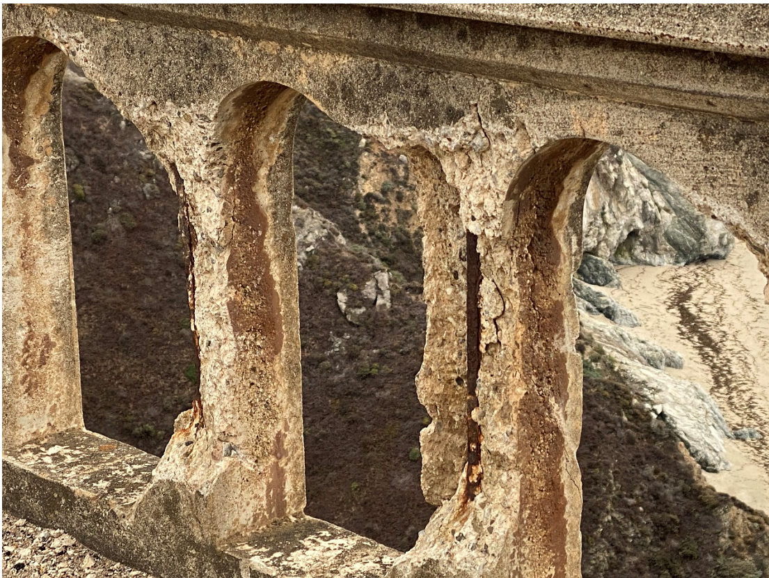
Figure 1-2 Photo of Bixby Creek Bridge Rail Deterioration
