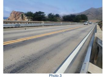
Thrie beam installation at the interior of both bridge rails (shown from Abut. 1, right).
