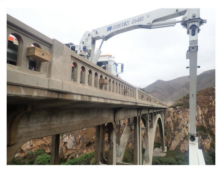
Photo No. 1 UBIT deployment off of the right side of structure (NB lane).
