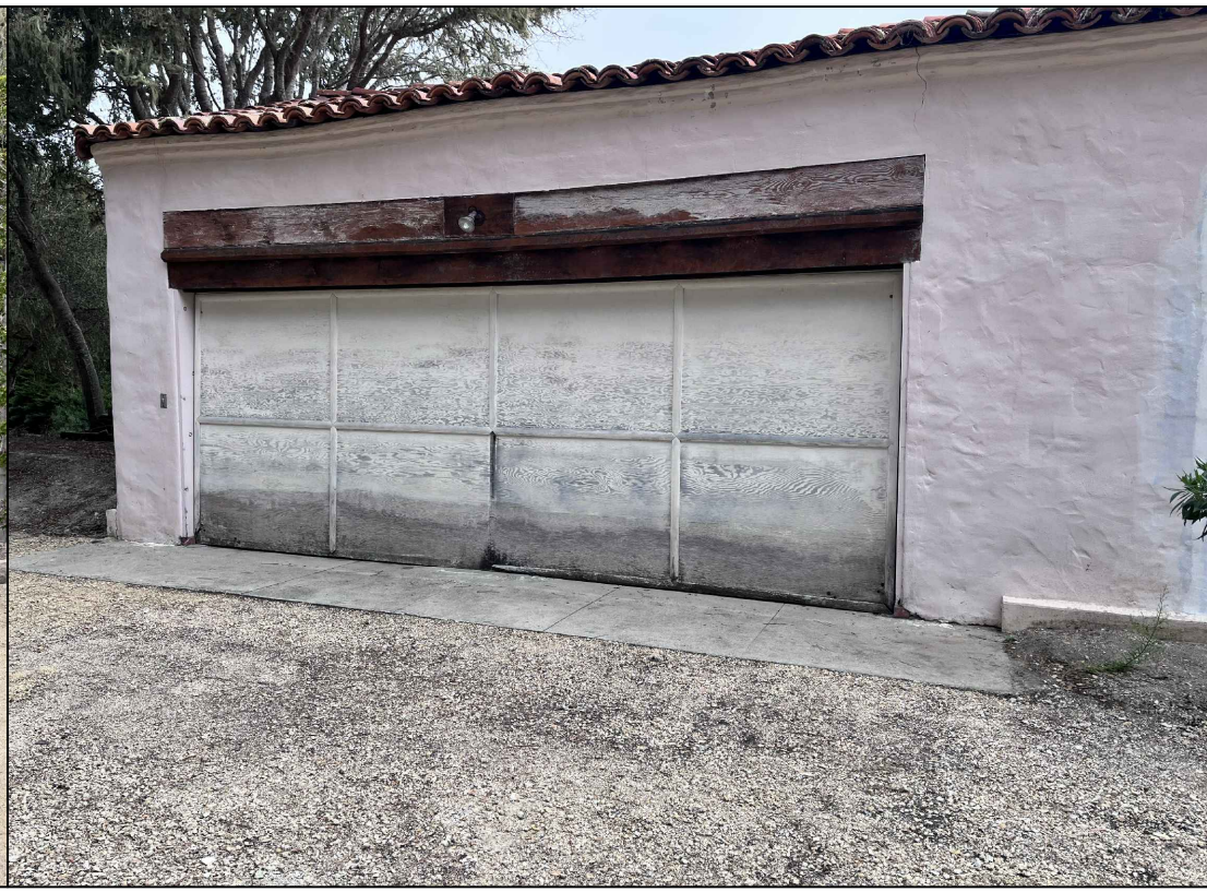
② GARAGE: REPAIR PREVIOUSLY ALTERED GARAGE DOOR OPENING W (N) WOOD DOORS. SEE (2) DOOR EXAMPLE TO THE RIGHT & A3.0.1 GARAGE DETAILS
