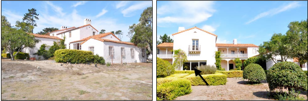
Figures 3 and 4. Left image shows the rear (south) and east elevations, showing the massing and arched chimneys. Right image details the rear (south) elevation. The living room windows (arrow) have been replaced with fixed glass.
