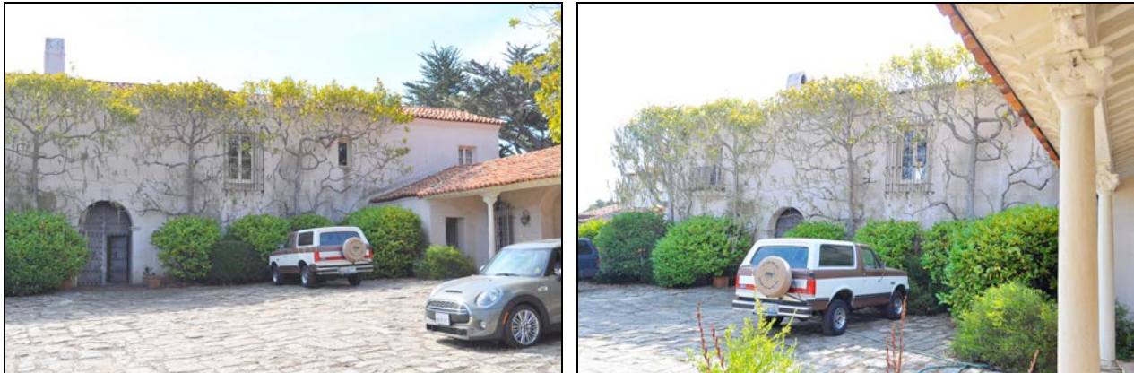
Figures 1 and 2. Left image shows the front (north) elevation. Carmel stone garden walls create a parking courtyard, with a garage wing on the west side. Right image shows the front elevation viewed from the garage wing.
