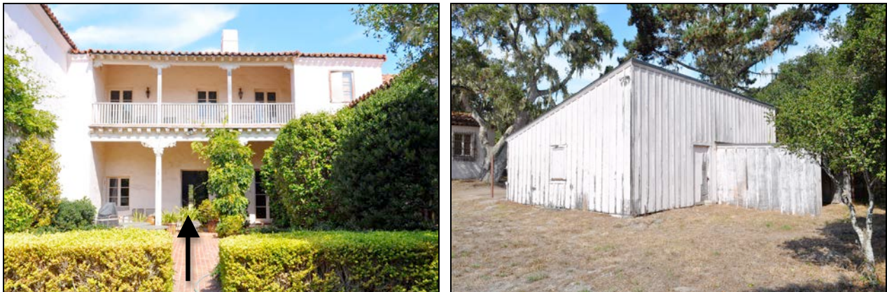
Figure 5. Left image details the rear-elevation arcade and terrace. A single pair of French doors has been replaced with fixed glass (arrow). Right image details the shed outbuilding.
