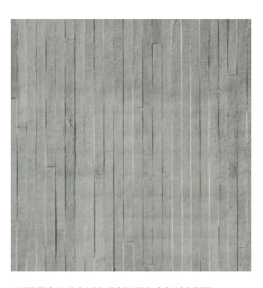
VERTICAL BOARD FORMED CONCRETE - RETAINING WALLS
