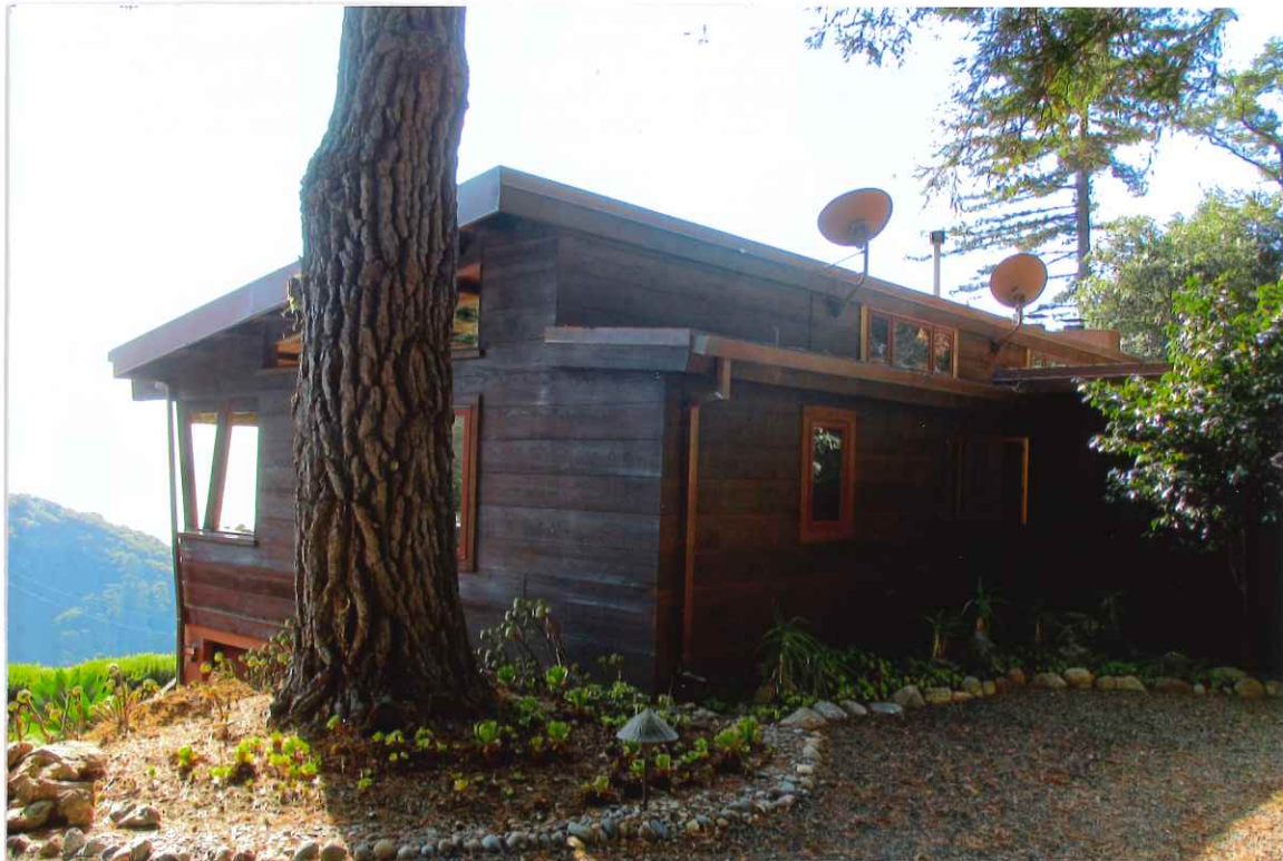
Photo #2. Looking SW at the East side-elevation. Note original lower bathroom & service spaces on the NW rear elevation. Kent Seavey, November, 2020.
