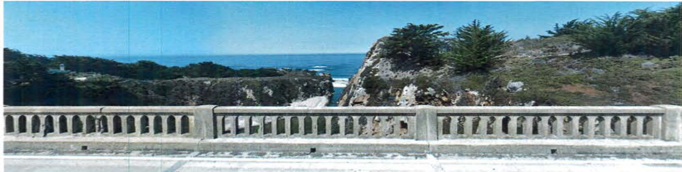
EXISTING ON DECK VIEW
