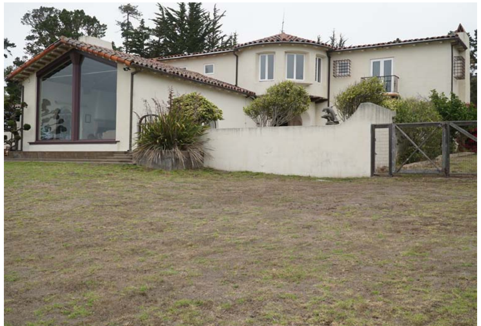
Figure 2. Looking northwest at south and east sides, 7/22/21.
