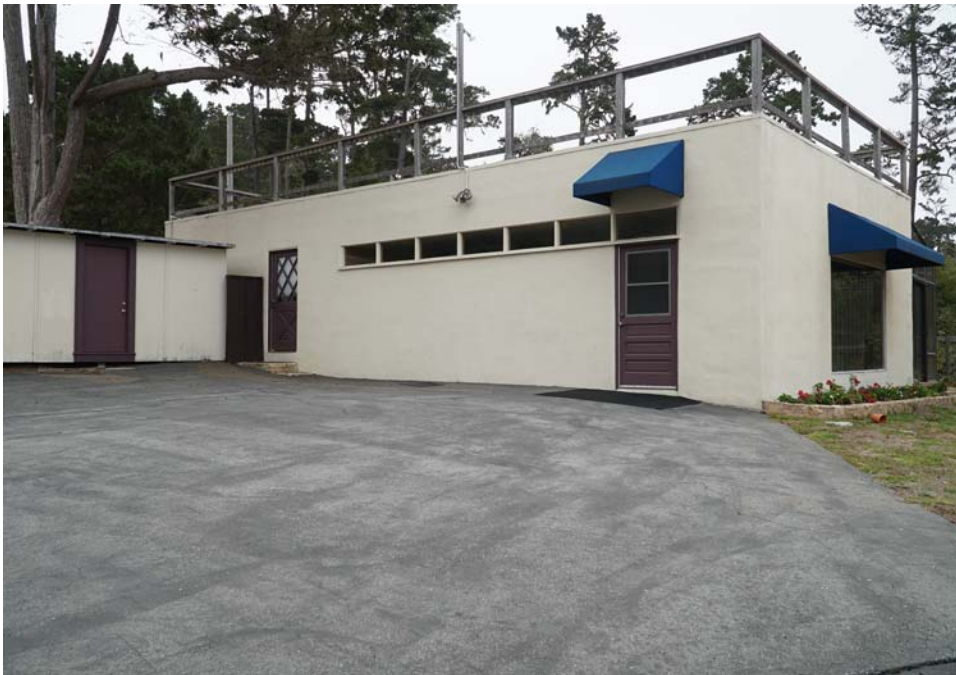
Figure 3. Looking northeast at west and south sides of servants' quarters, game room/green house, 7/22/21.
