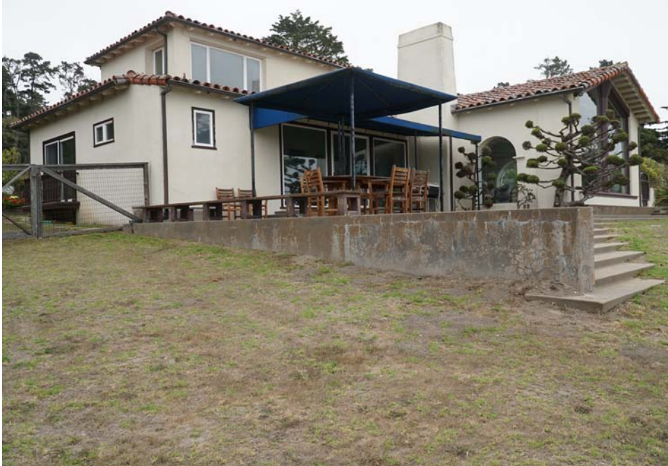
Figure 1. Looking northeast at west and south sides, 7/22/21.
