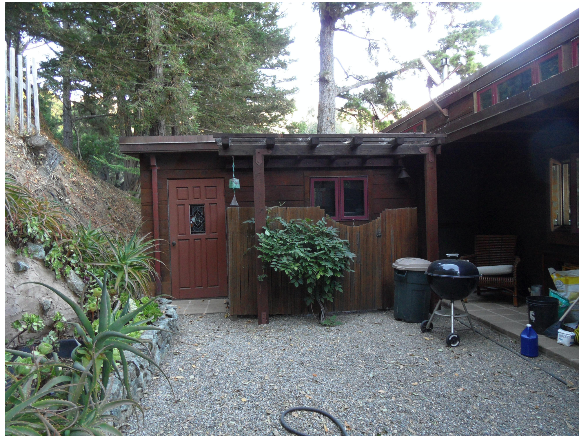
NON-HISTORIC ADDITION TO BE REMOVED
