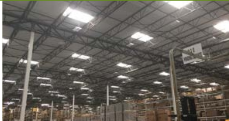
PHOTO: A combination of natural and LED lights provide the right mix of lighting sources
