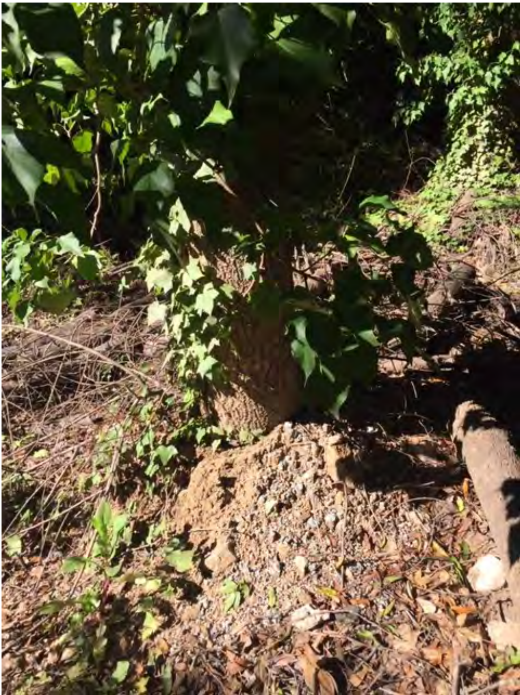
Figure 11. One of a few examples where fill material is smothering the lower trunk and root crown of roadside trees.
