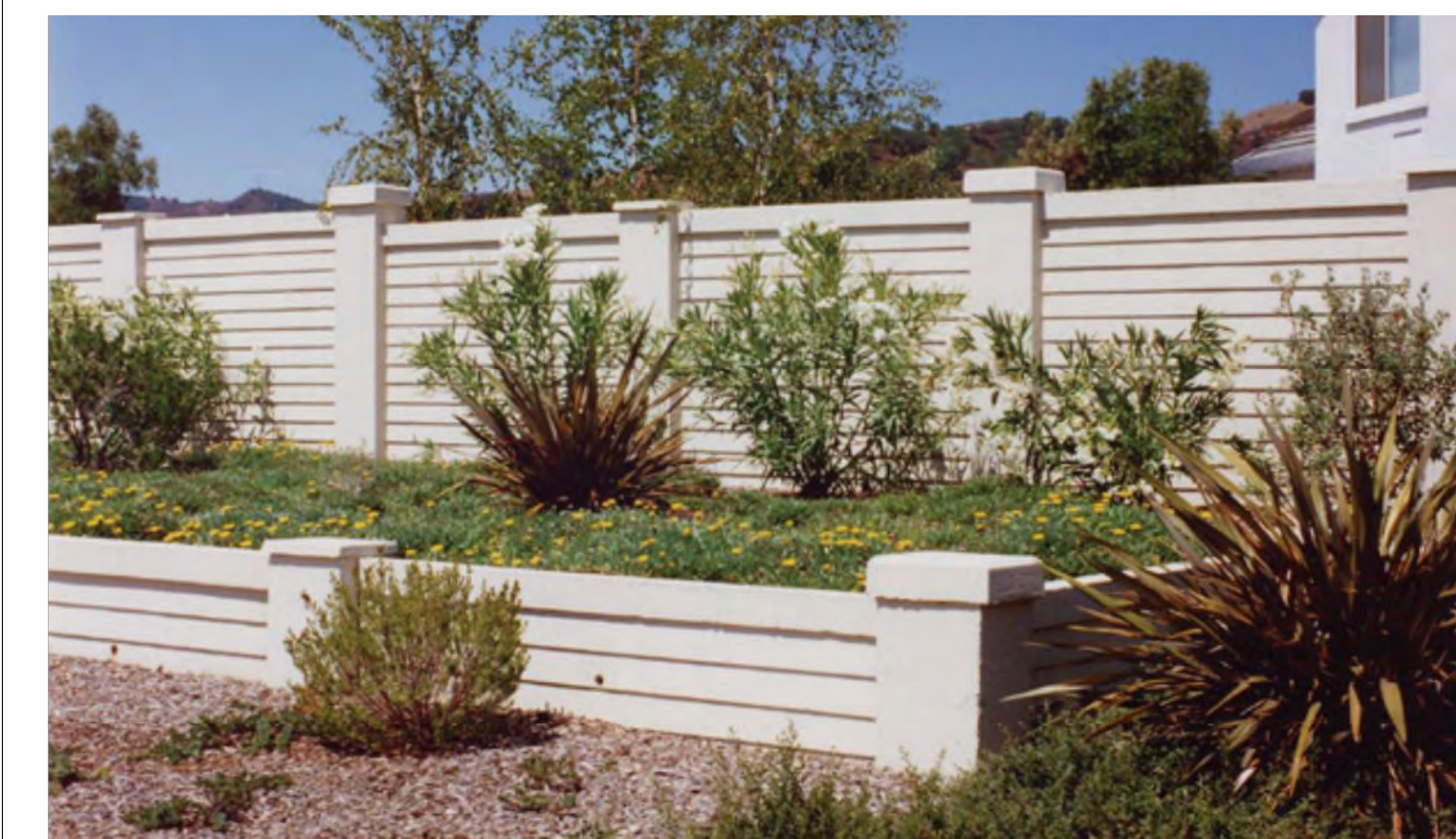
4 8'-0" HIGH PRECAST CONC. WALL OLDCASTLE - SIERRA WALL SYSTEMS "SHIPLAP" NOT TO SCALE
