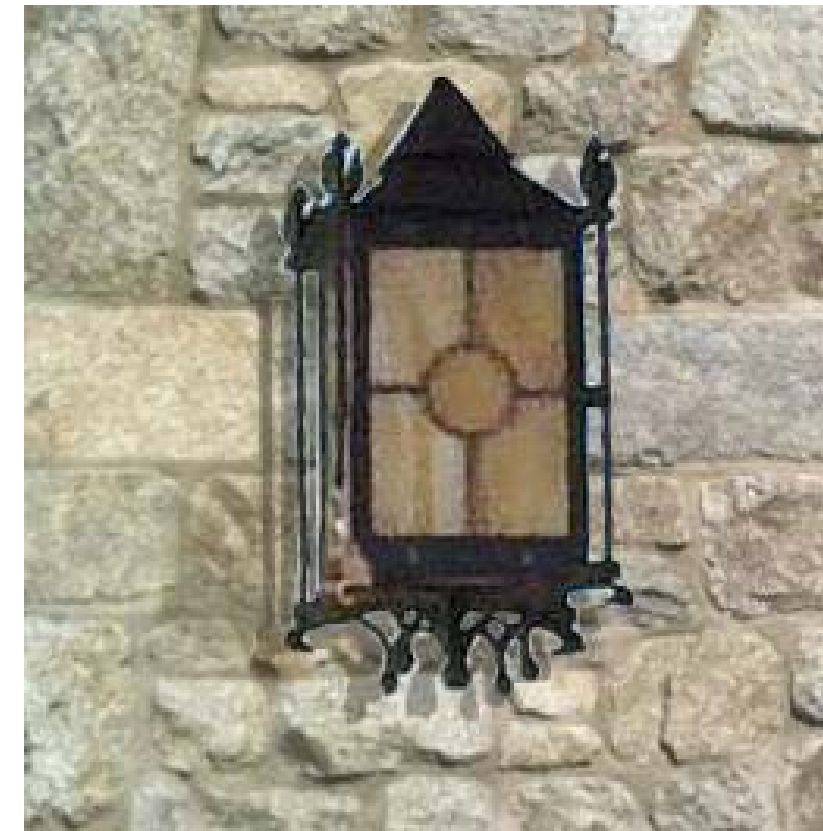
WALL SCONCES AT EXTERIOR DOORS ON MAIN LEVEL, APPROX. 35 WATTS EA.
