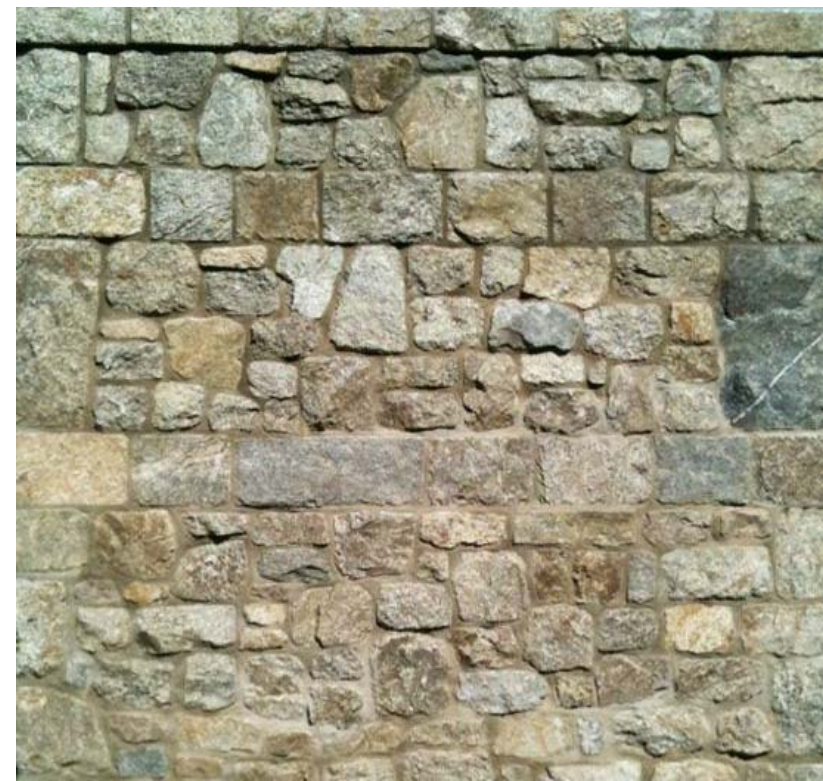
GRANITE ROCK WALL
