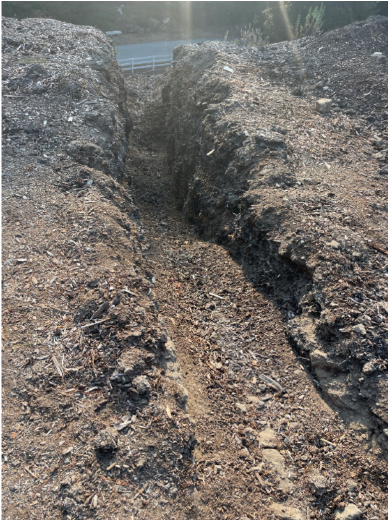
Exploratory digs have an accumulation of approximately 12 feet in depth with excessive buildup around trees that will have to be removed manually to minimize impacts.
