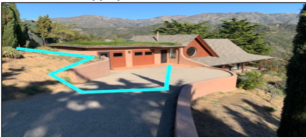
Proposed geothermal location in driveway.
