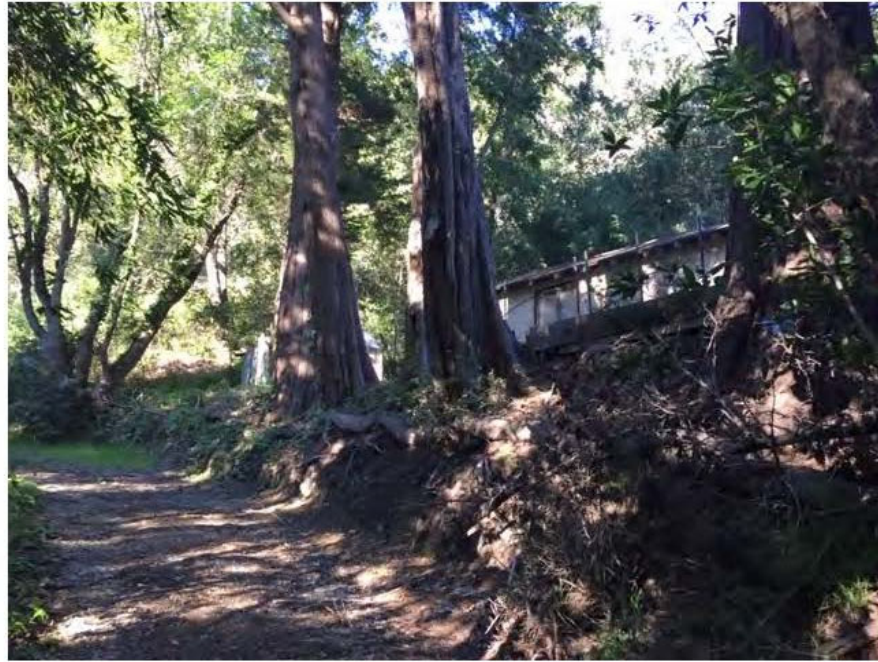
Figure 9. Blaze Engineering apparently cut in this non-permitted road just below the Donaldson's cabin, which resulted in several large roots being cut and damaged on the upper cut slope. This area is located just above the proposed office building.
