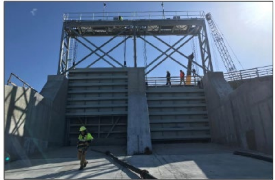
Upper Salmon Dam Gated Spillway
