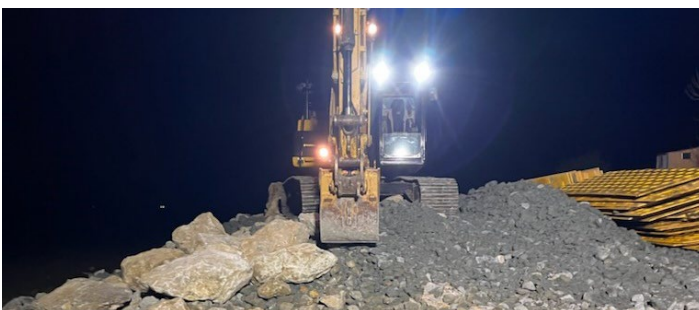
Debris Removal MCPW, CalTrans
