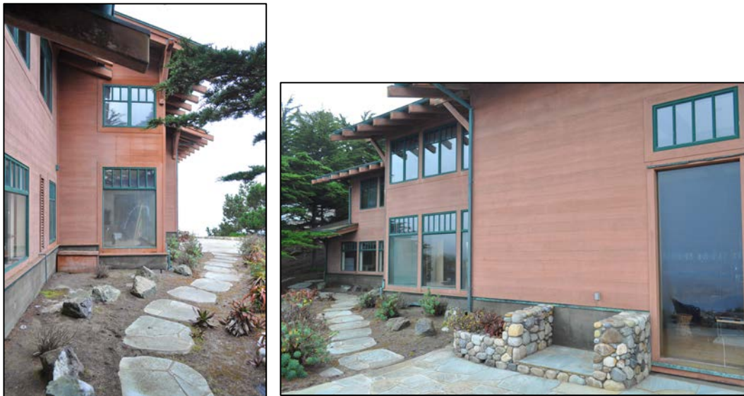
Figures 5 and 6. Left image details the north elevation looking northwest, showing the modern concrete foundation and windows installed in 1990. Right image details the north elevation looking southeast. All materials were installed onto the building during the extensive 1990 remodeling campaign.
