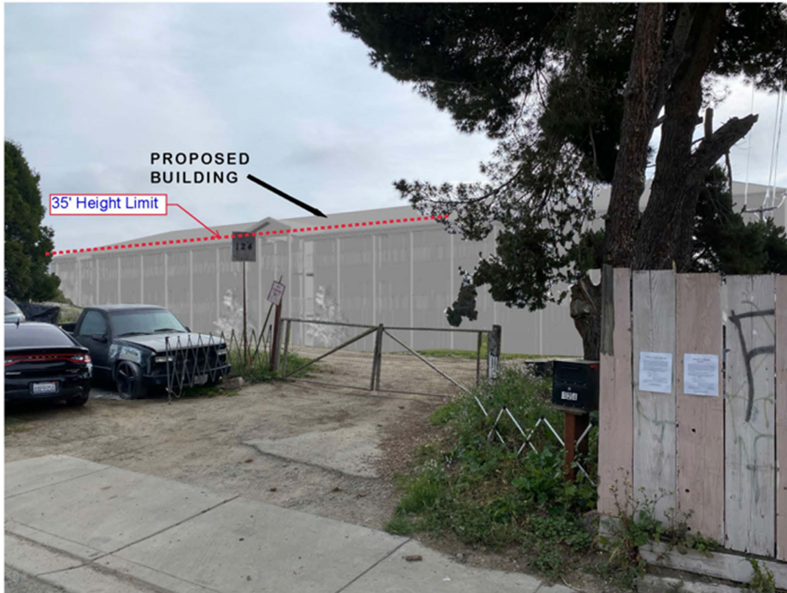
Figure 6. 3D modeled image captures the height of the proposed development buildings when viewed from street level at the driveway on Gonda Street. From this angle, the proposed buildings do not appear significantly taller than the 35-foot height maximum that is the
