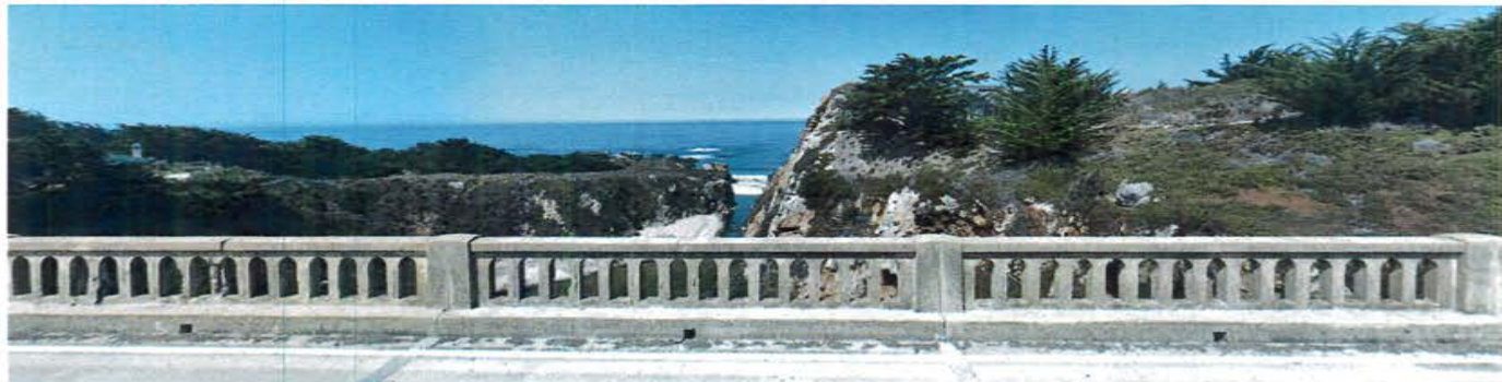
EXISTING ON DECK VIEW
