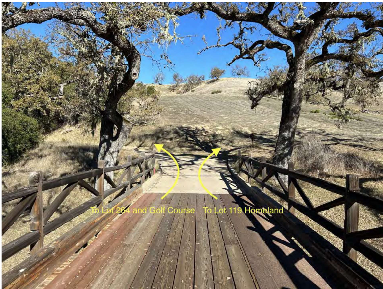
FIGURE 3. PHOTO OF LOT 119'S ACCESS ROUTE.
