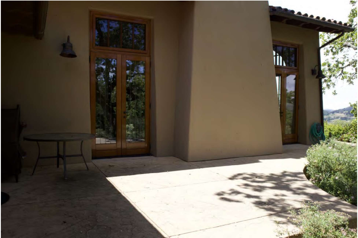
FIGURE 10. EXAMPLE OF BENEFICIAL USE OF HARDSCAPE AS PART OF THE NON-COMBUSTIBLE ZONE, AND FIRE-SAFE LANDSCAPING (PHOTO NOT OF LOT 119).
