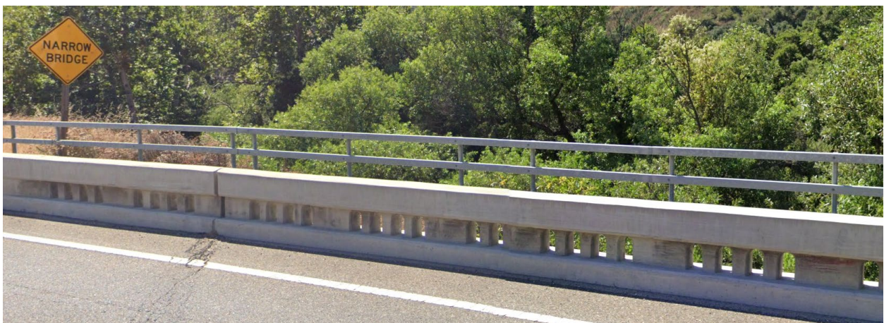
Figure 10: Type 80 Bridge Rails along Nojoqui Creek Corridor (Google Maps Imagery, May 2023)
