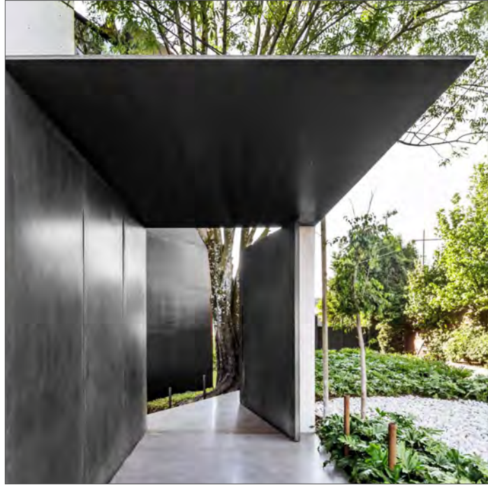
6 GREY PATINAED STEEL PLATE CANOPY, FINISH TO MATCH ADJ. ROOF FASCIA
