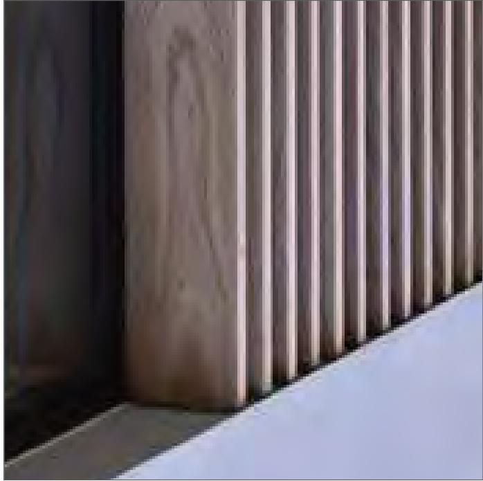
5 VERTICAL WD. SCREEN OVER WINDOW SYSTEM - 2x WD. MEMBERS; SPECIES TBD; LIGHT/NATURAL FINISH
