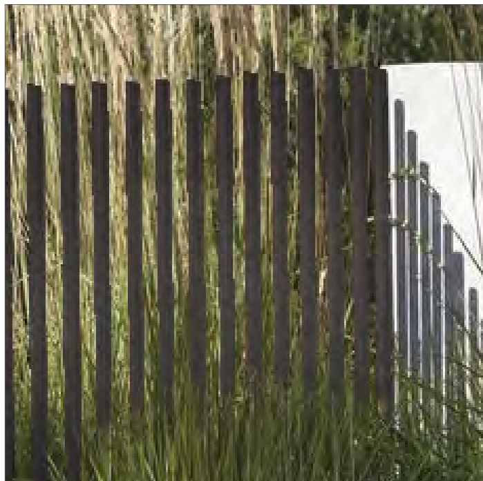
8 CIRCULAR 1.5" DIAM. WD. ROD FENCE & ENTRY DECK GUARDRAIL, 3" O.C. SPACING, ATTACHED TO CONCRETE CURB FOOTING
