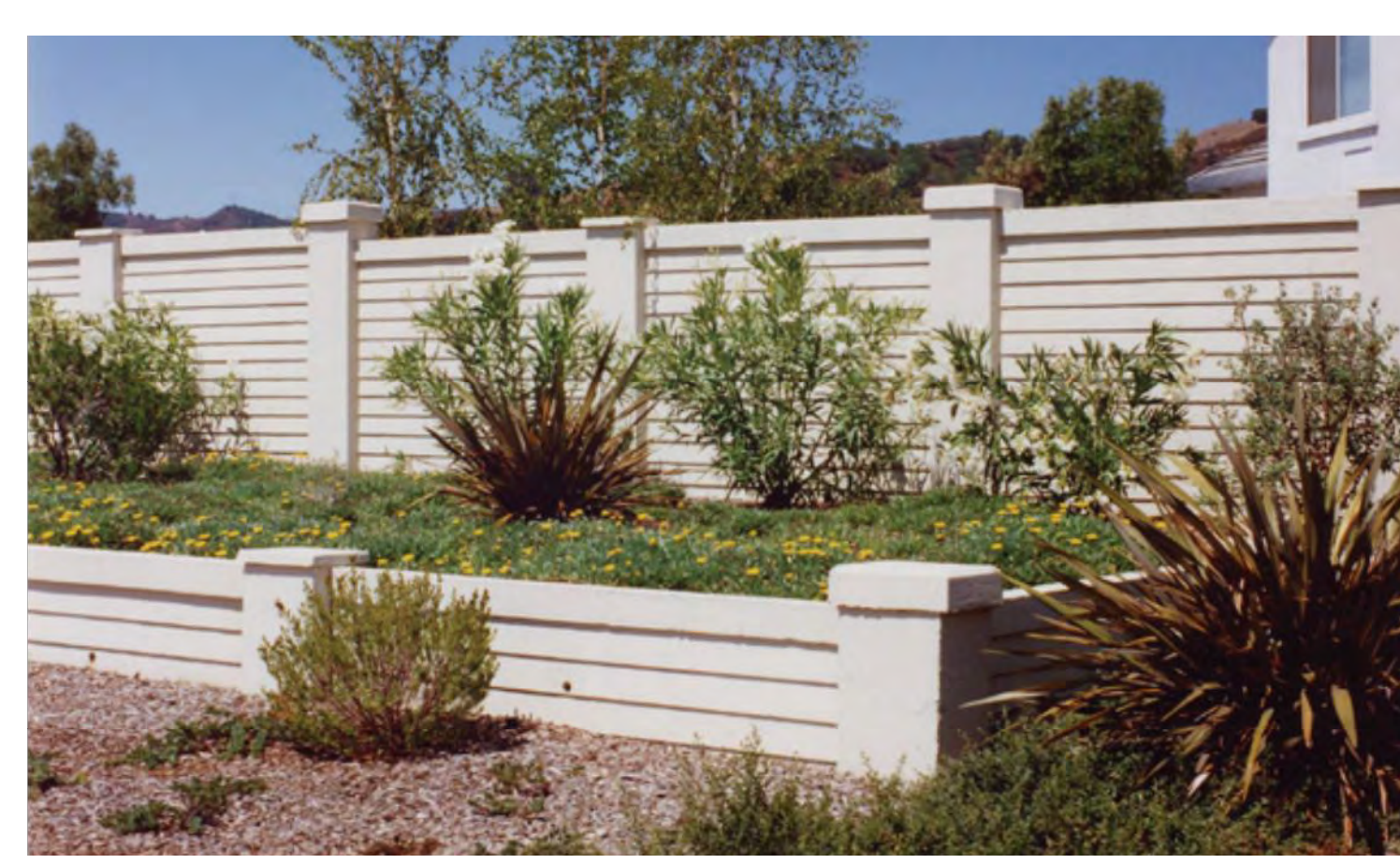
4 8'-0" HIGH PRECAST CONC. WALL OLDCASTLE - SIERRA WALL SYSTEMS "SHIPLAP" NOT TO SCALE
