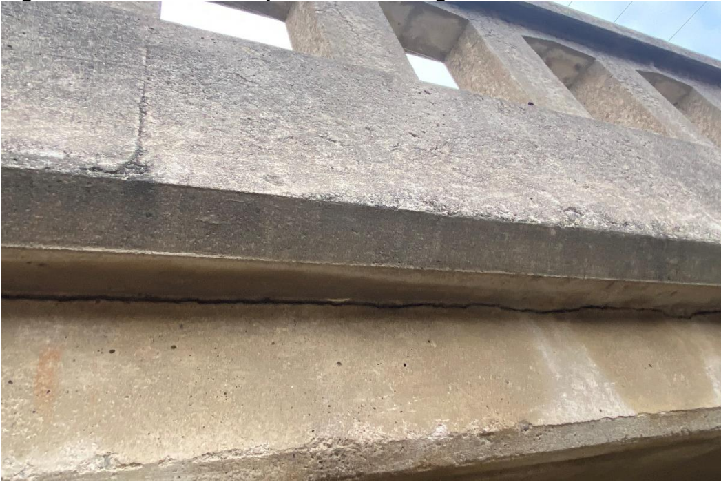
Figure 1-7 Photo of Malpas Creek Bridge Rail Deterioration
