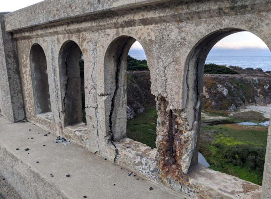
Figure 1-4 Photo of Garrapata Creek Bridge Rail Damage
