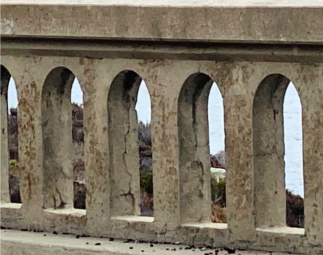
Figure 1-7 Photo of Malpas Creek Bridge Rail Deterioration
