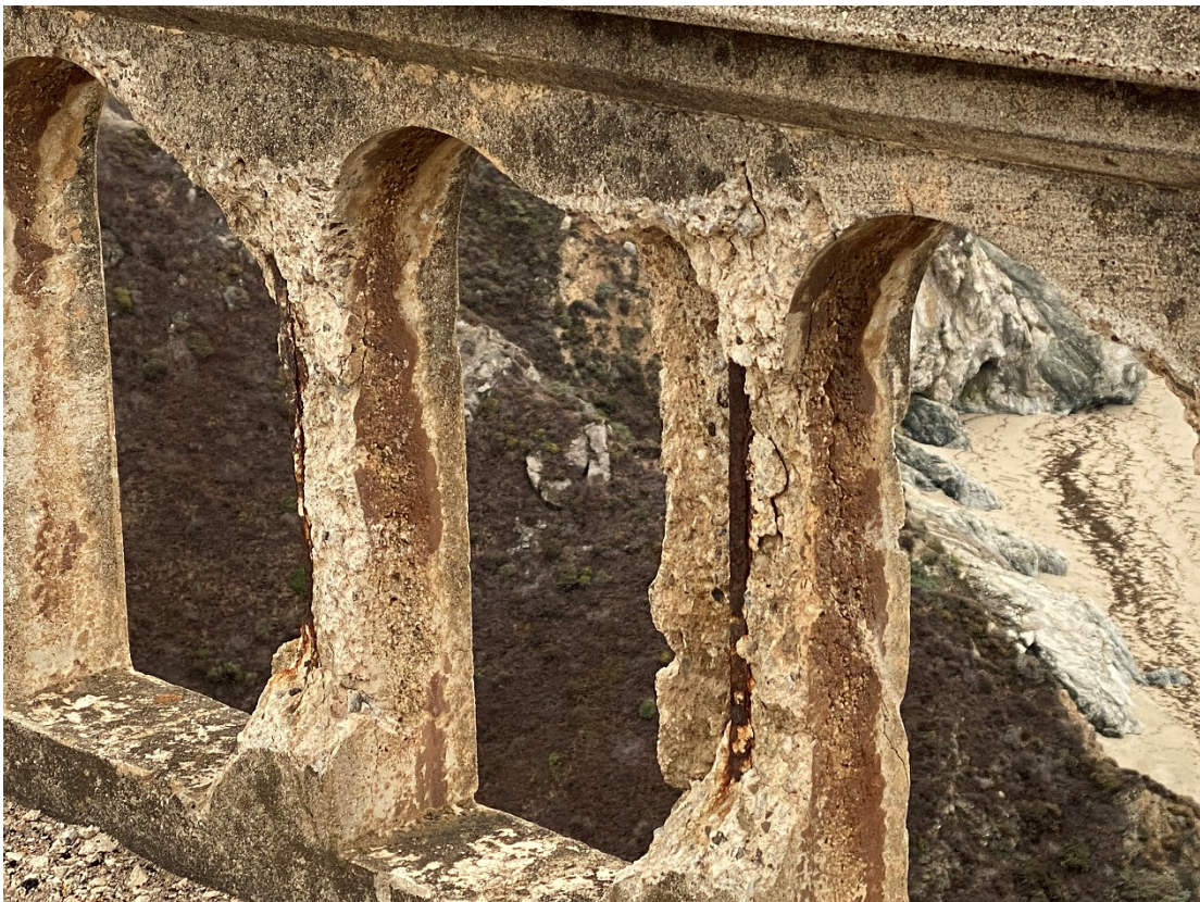
Figure 1-2 Photo of Bixby Creek Bridge Rail Deterioration
