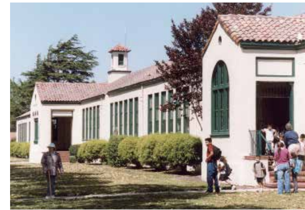
Even single-story buildings, when symmetrically arranged, can have a significant community presence.
