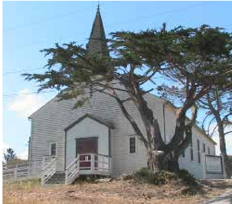
Front facade of the Chapel
