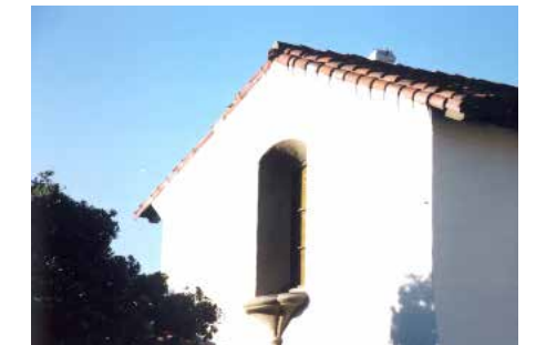
Flush face at rake focuses attention on the elevation.
