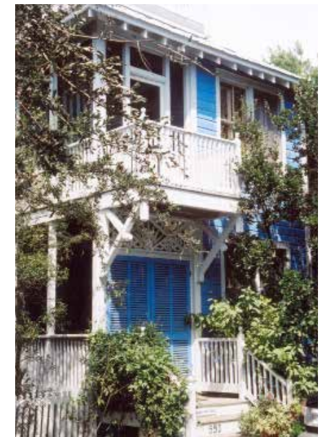
Craftsman porch details are structurally expressive.
