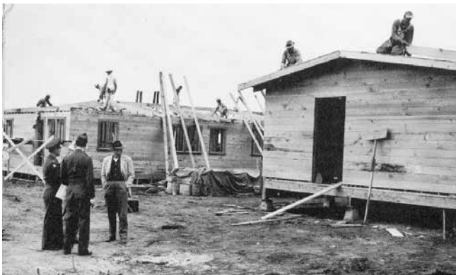
Figure 2.24 Construction at East Garrison circa 1940
