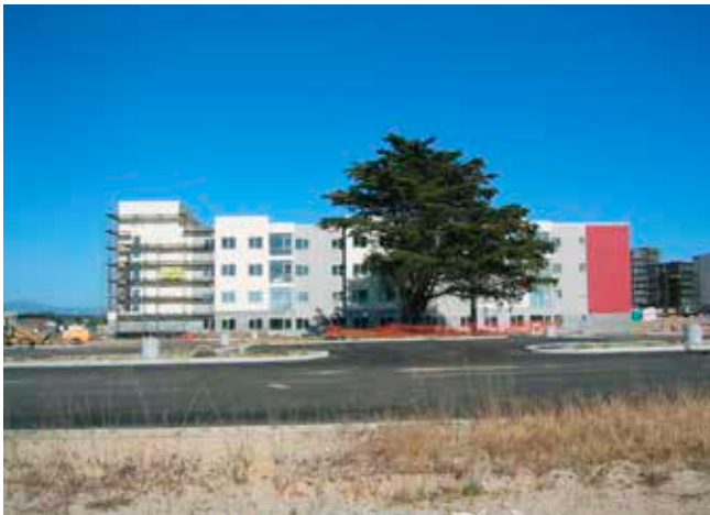
Figure 3.19 New construction at CSUMB
