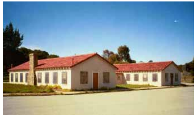
Figure 2.26 WPA-built mess hall
