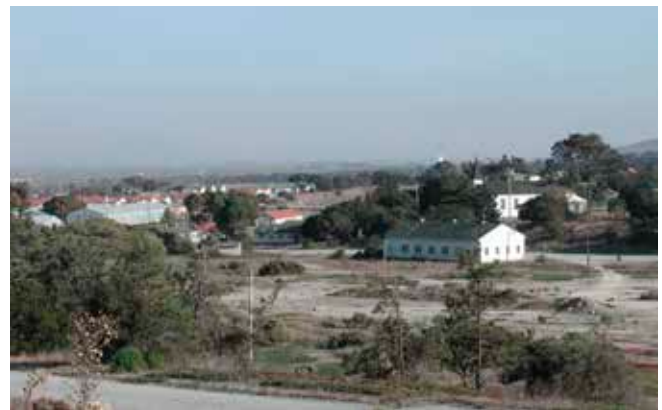
Figure 1.4 Abandoned buildings at East Garrison
