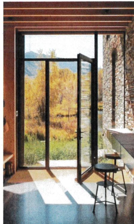
ALUM. FRAME, HINGED DOOR AND SAME FOR FRENCH DOORS
