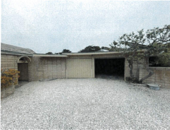
GARAGE FROM PARKING AREA
