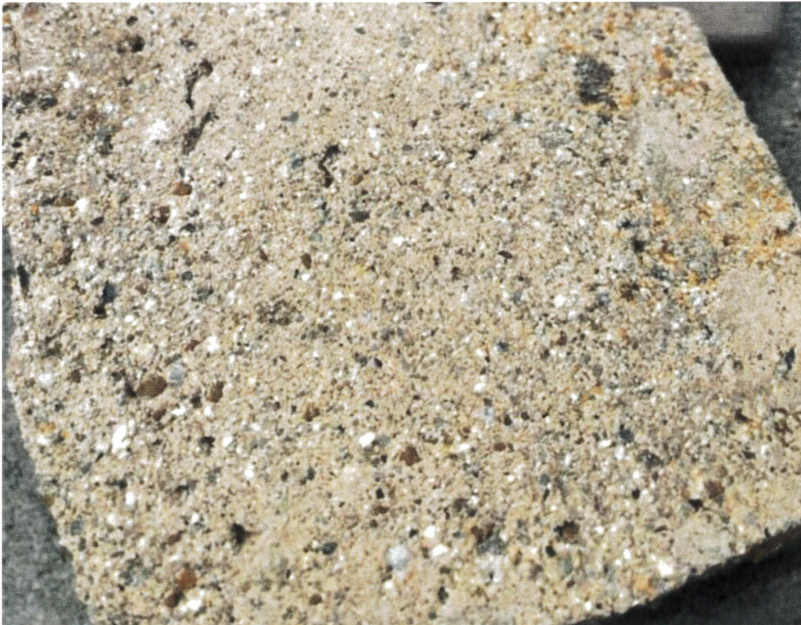
EXISTING WALLS: TAN CONCRETE SLUMP STONE BLOCK
