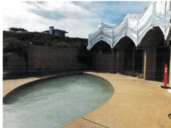
COURTYARD VIEW – GARAGE NORTH WALL
