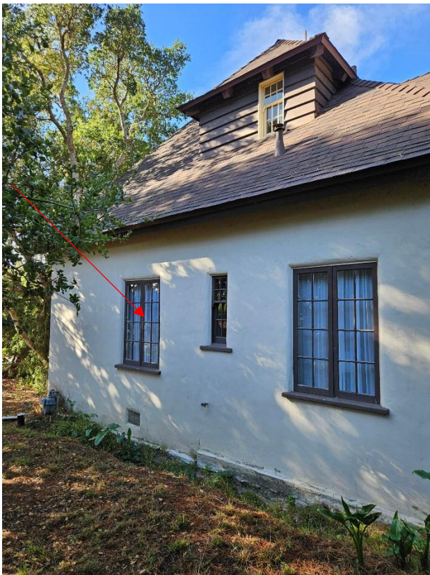
Figure 3: View of east elevation. The arrow indicates the window that will be moved to the left and replaced with a door.
