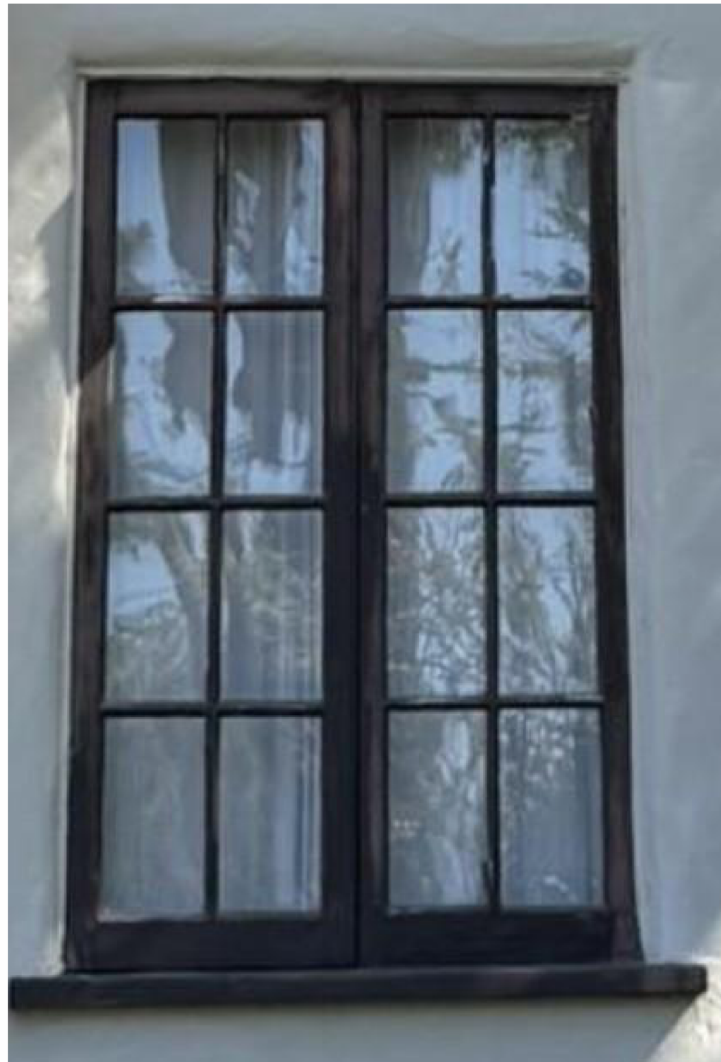
PROPOSED WINDOW TYPE ( MATCH ( E ) AT EXISTING AND ALUMINUM CLAD AT THE NEW ADDITION/ REMODEL
