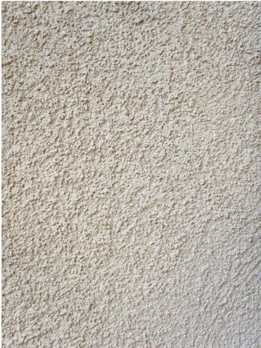
EXTERIOR SITE WALLS: STUCCO OVER CONCRETE
