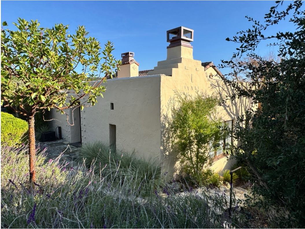
Figure 24. North and west elevations, facing southeast.
