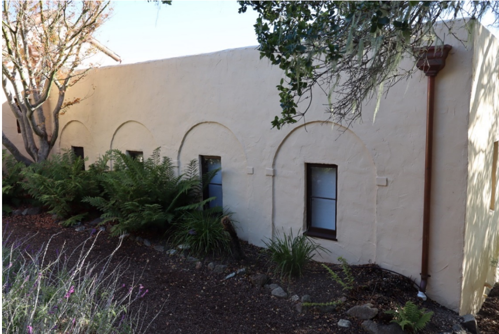
Figure 10. Blind arcade on the west wing of the north elevation, facing southeast.
