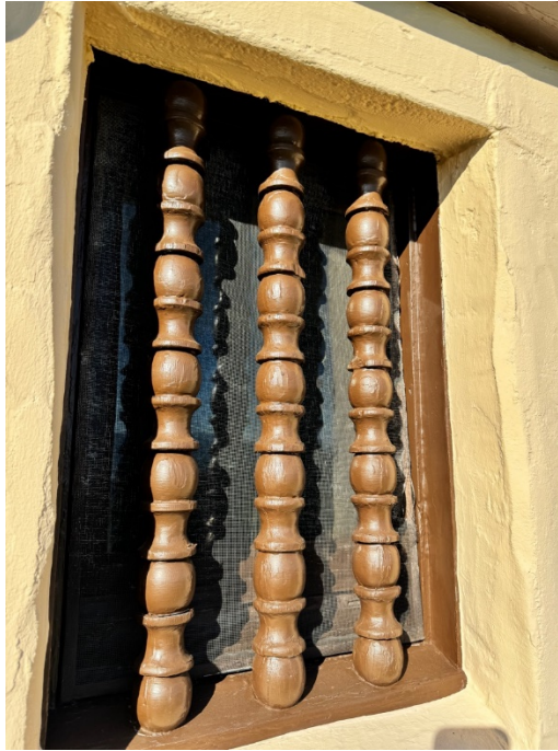
Figure 19. Wood grille within window of blind arcade on south elevation.
