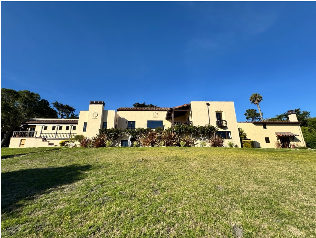
Figure 32. South elevation, facing north.
