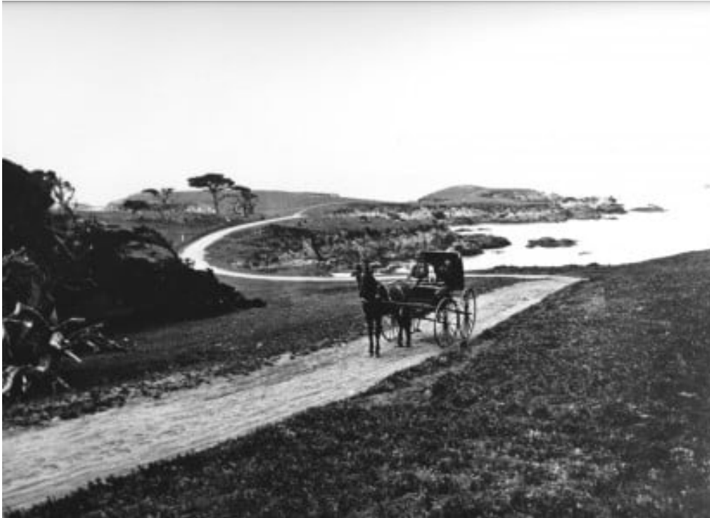
Figure 5. ca. 1881 photograph of 17-Mile Drive in Pebble Beach, and a section known as the loop (courtesy of 2025 Pebble Beach Company).
