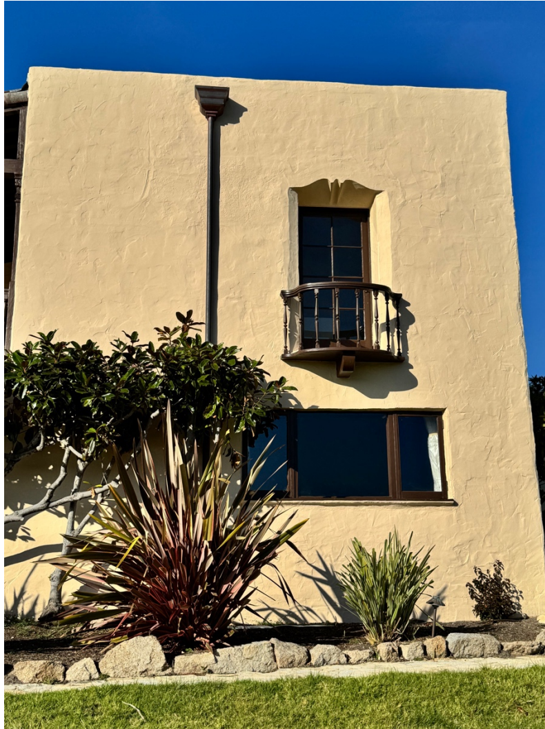
Figure 63. Eight-light wood door set within a decorative alcove with Juliet balcony above picture window, facing north.
