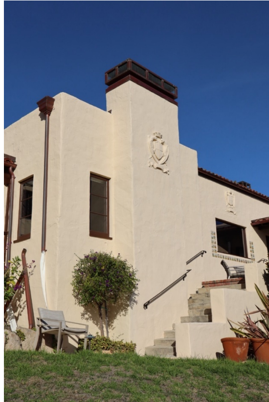
Figure 35. Exterior stucco chimney and steps leading to rear, raised patio, facing northeast.
