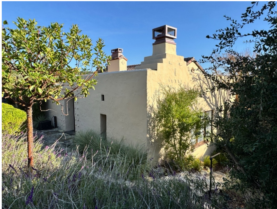
Figure 9. North and west elevations, facing southeast.
