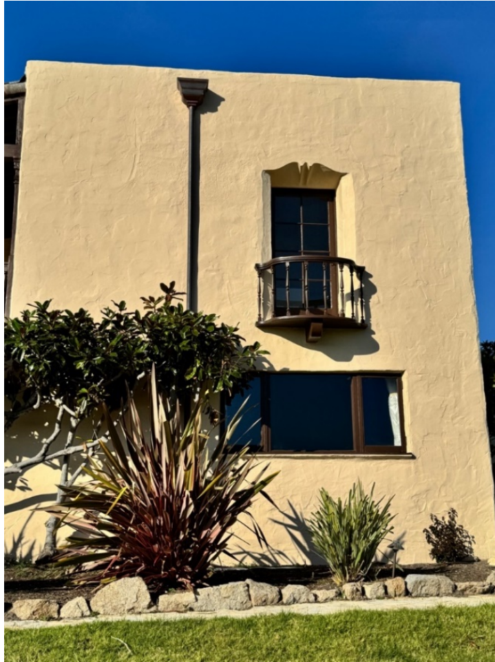
Figure 61. Eight-light wood door set within a decorative alcove with Juliet balcony above picture window, facing north.
