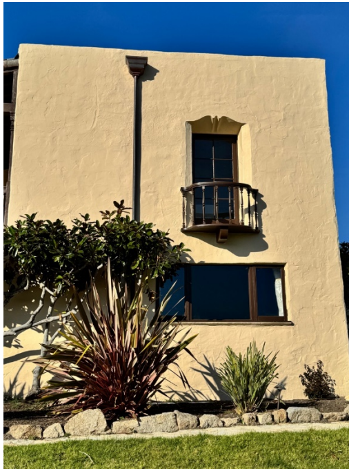
Figure 28. Eight-light wood door set within a decorative alcove with Juliet balcony above picture window, facing north.
