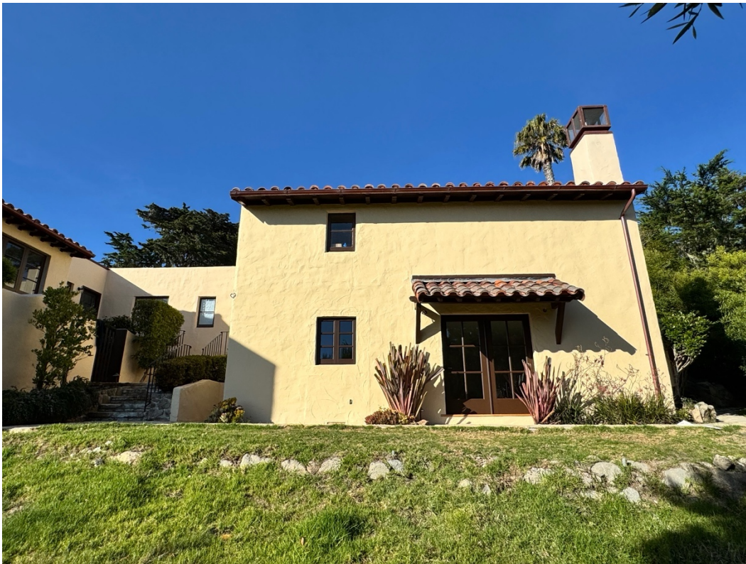
Figure 37. South elevation, facing north.
