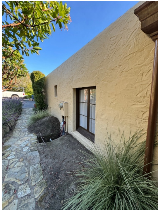
Figure 19. East wing of north elevation, facing southeast.
