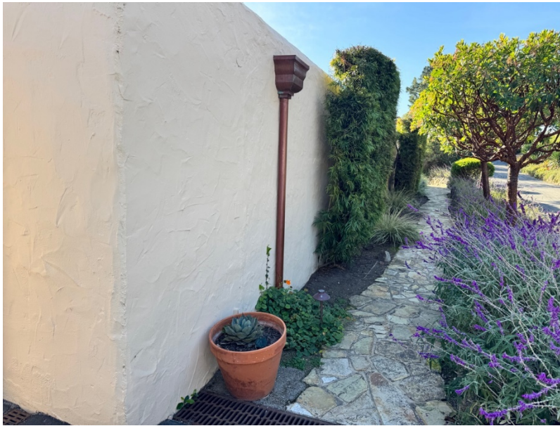
Figure 2. East wing of north elevation, facing southwest.
