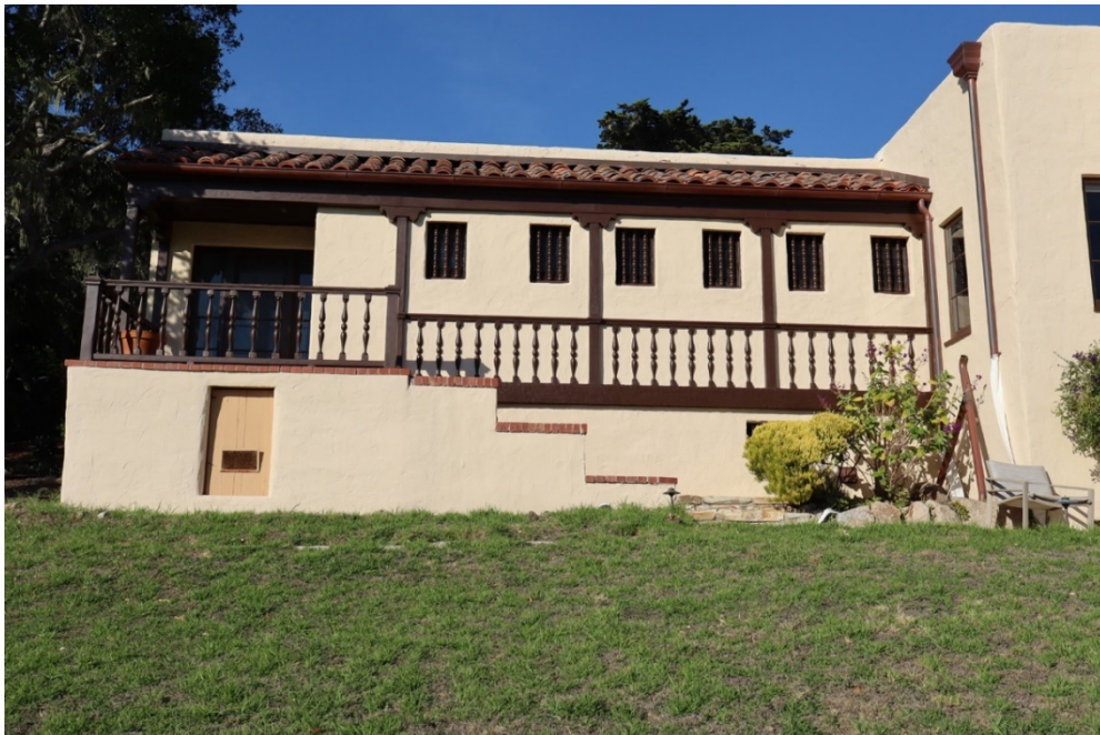
Figure 18. Blind colonnade on the west elevation of the south elevation, facing north.
