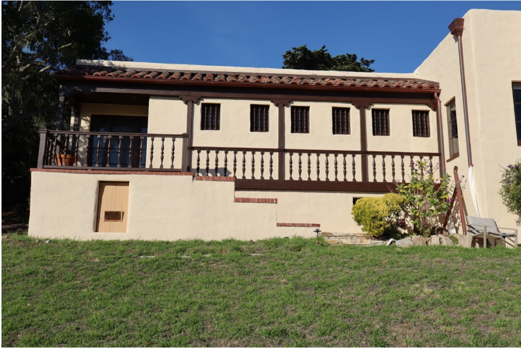
Figure 33. Blind colonnade on the west elevation of the south elevation, facing north.
