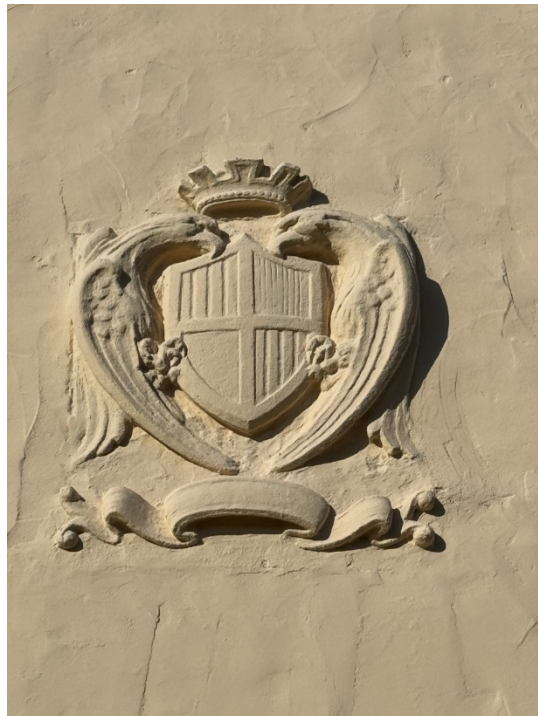
Figure 22. Stucco cartouche on exterior stucco chimney of the south elevation.
