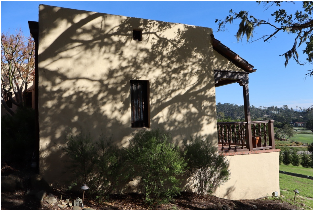
Figure 47. West elevation of west wing, facing east.
