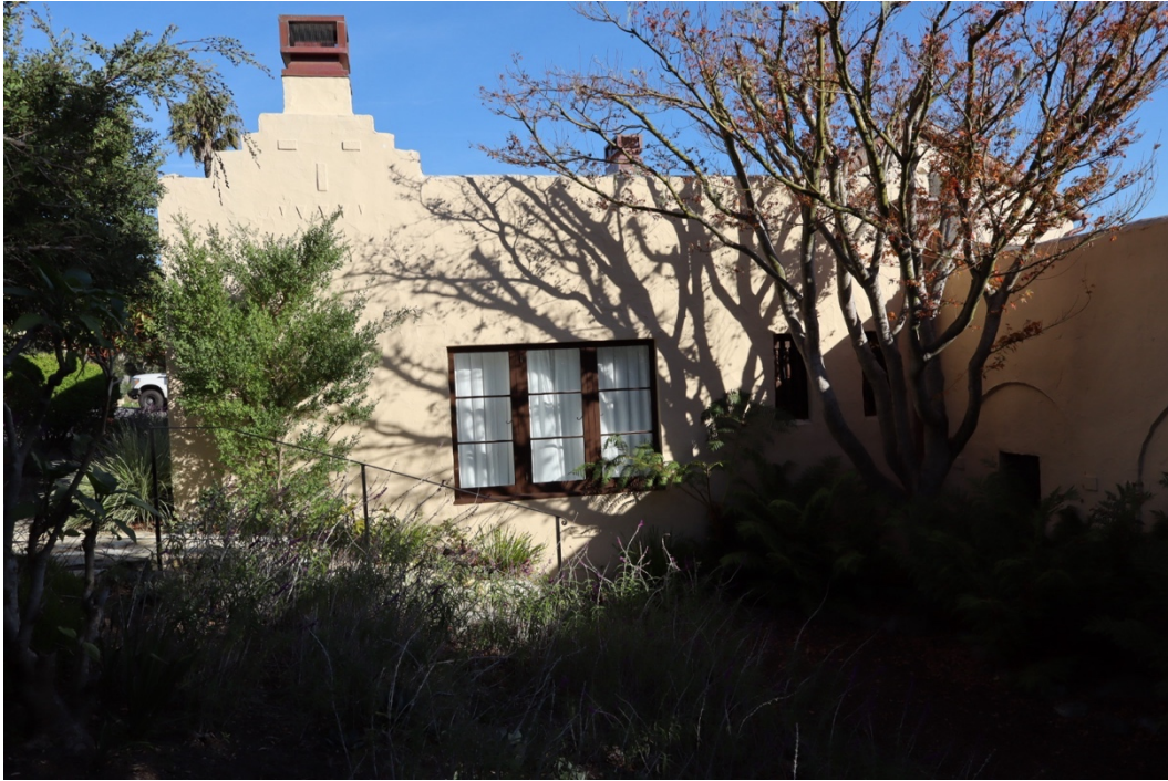
Figure 46. West elevation with stepped parapet to stucco chimney, facing east.
