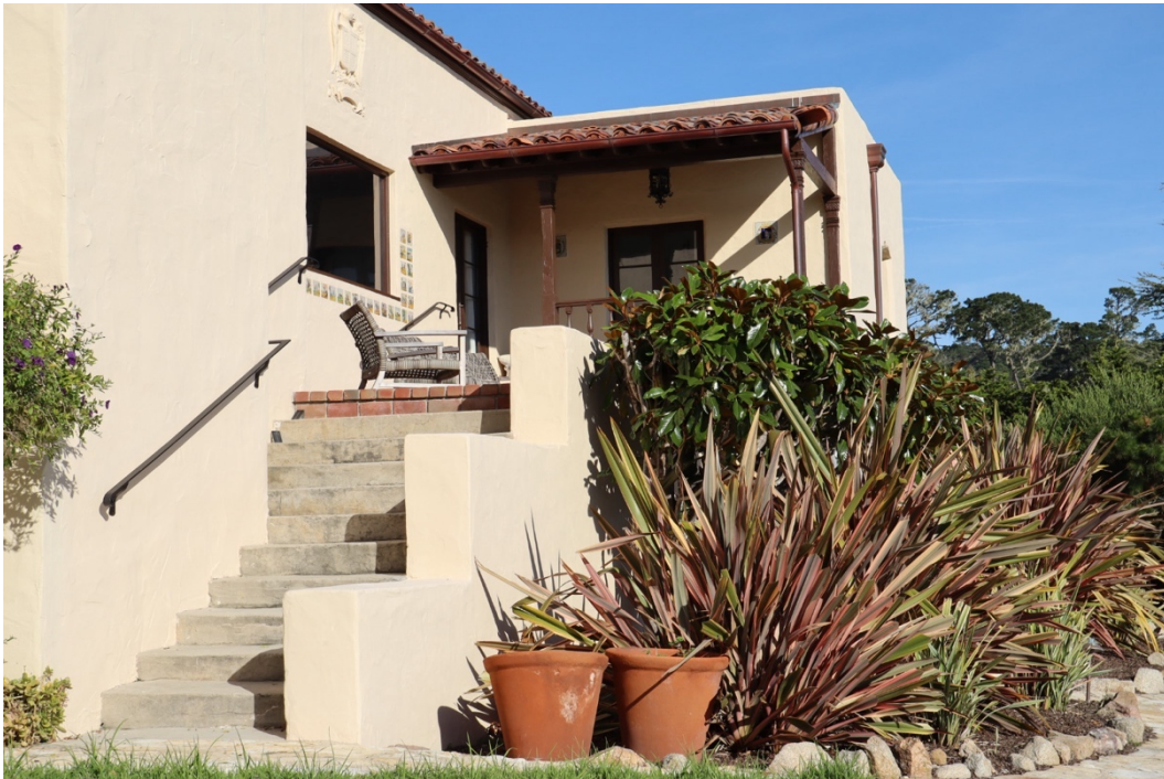
Figure 49. West elevation within the rear patio, facing northeast.
