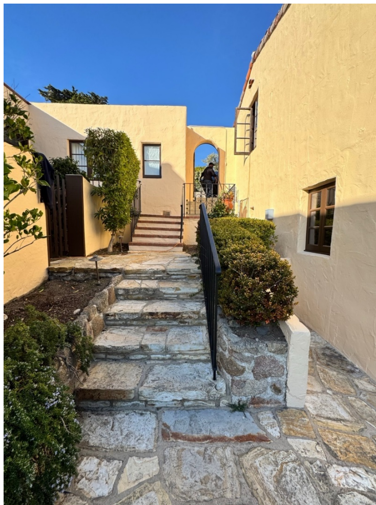
Figure 65. South elevation of the east wing, with wing wall, connected the 1920 house to ca. 1930 garage, facing north.
