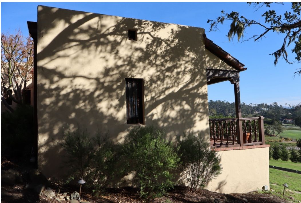
Figure 32. West elevation of west wing, facing east.
