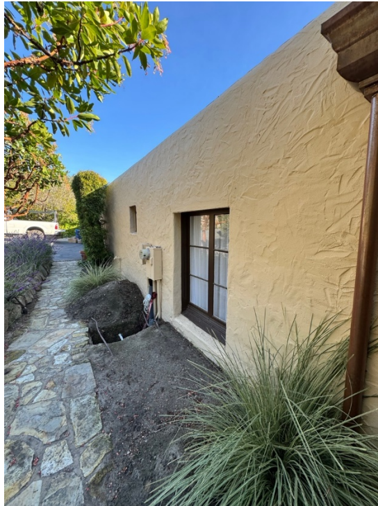
Figure 4. East wing of north elevation, facing southeast.
