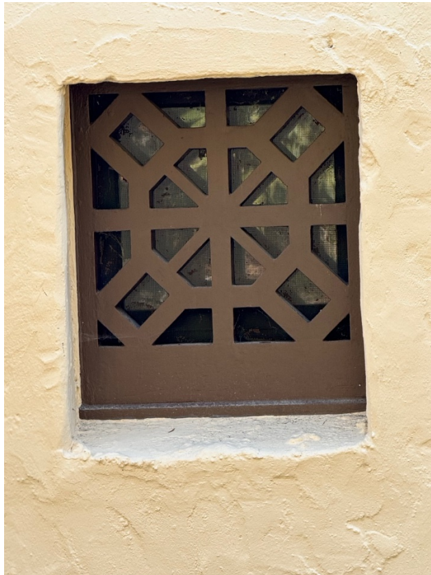
Figure 3. Detail of geometric wood grille.
