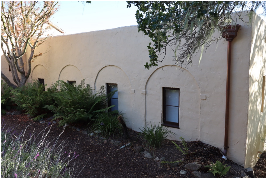
Figure 25. Blind arcade on west wing of the north elevation, facing southeast.
