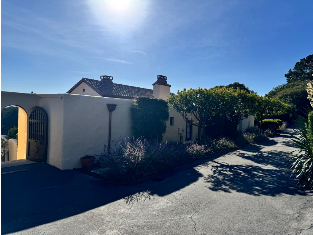
Figure 16. North elevation, facing southwest.
