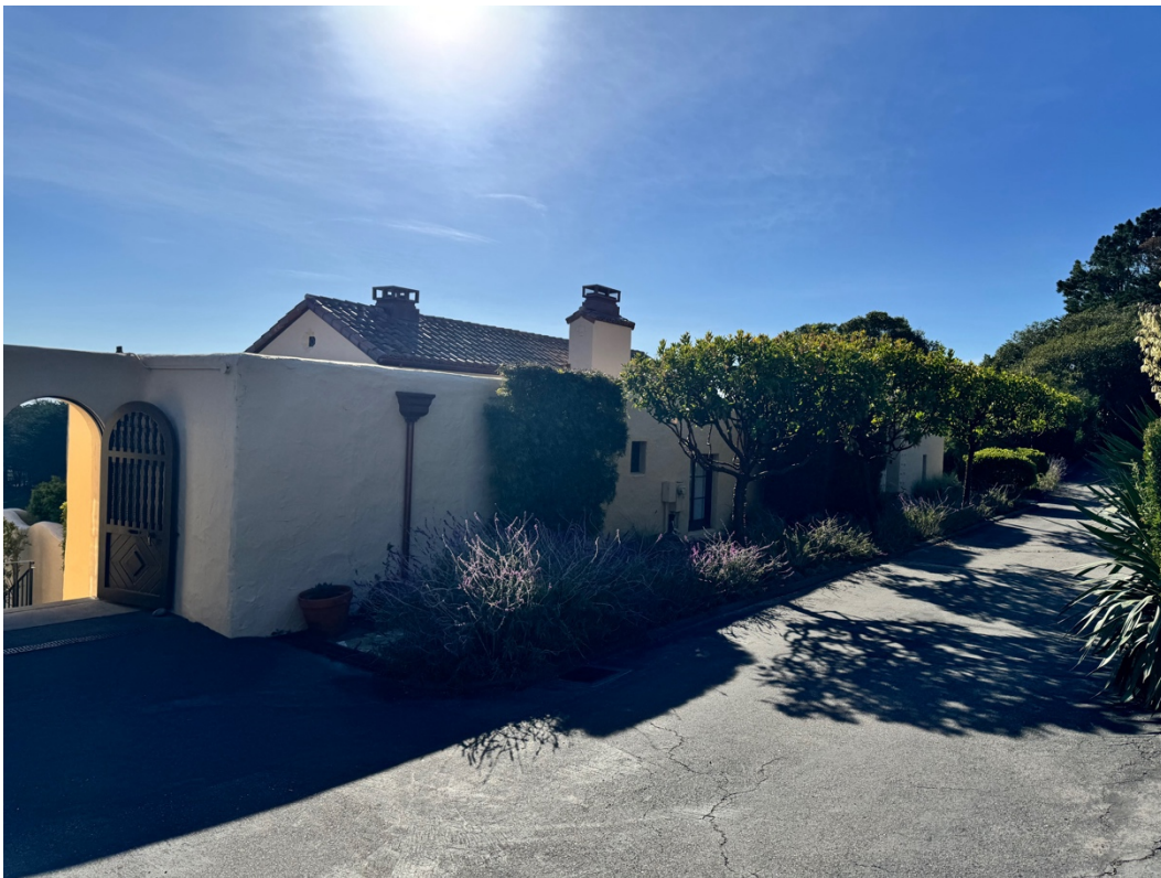
Figure 1. North elevation, facing southwest.
