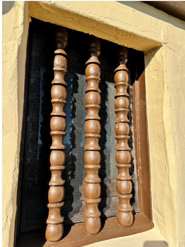
Figure 34. Wood grille within the window of the blind arcade on the south elevation.
