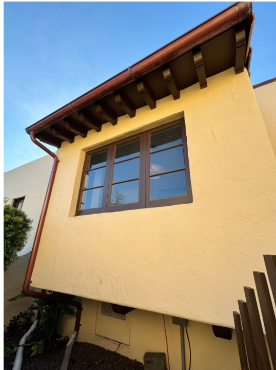
Figure 13. Projecting bay window on the east elevation, facing southwest.
