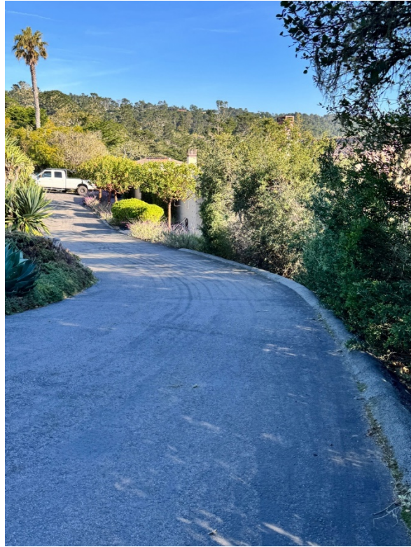
Figure 54. Driveway along the north elevation of the 1920 house.
