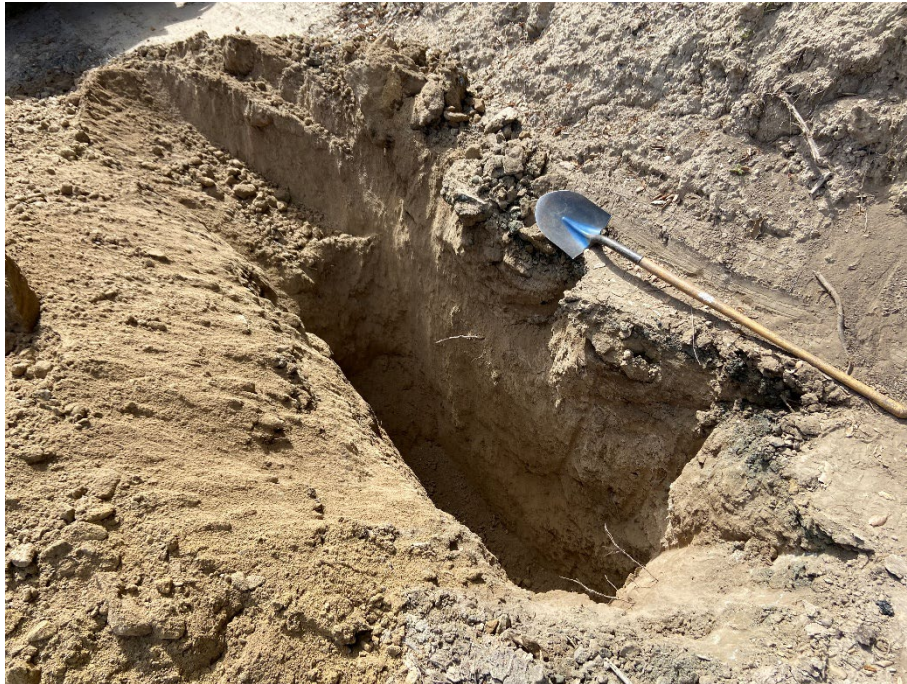
Photo #3: Excavation of TP-1, Artificial Fill Zone
