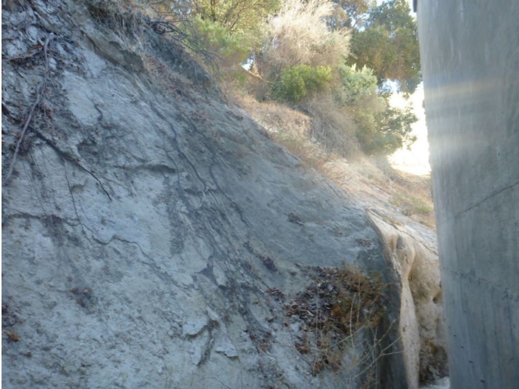
Photograph 8. Red bluffs behind Powerhouse. The roots on the failure surface.
