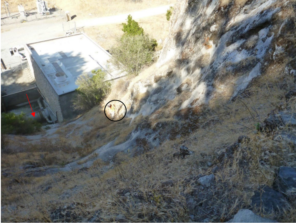
019 Photograph 2 looking down debris flow from access road . Note exposed pentstock in middle of (arrow) and geobags (circled) for sale.
