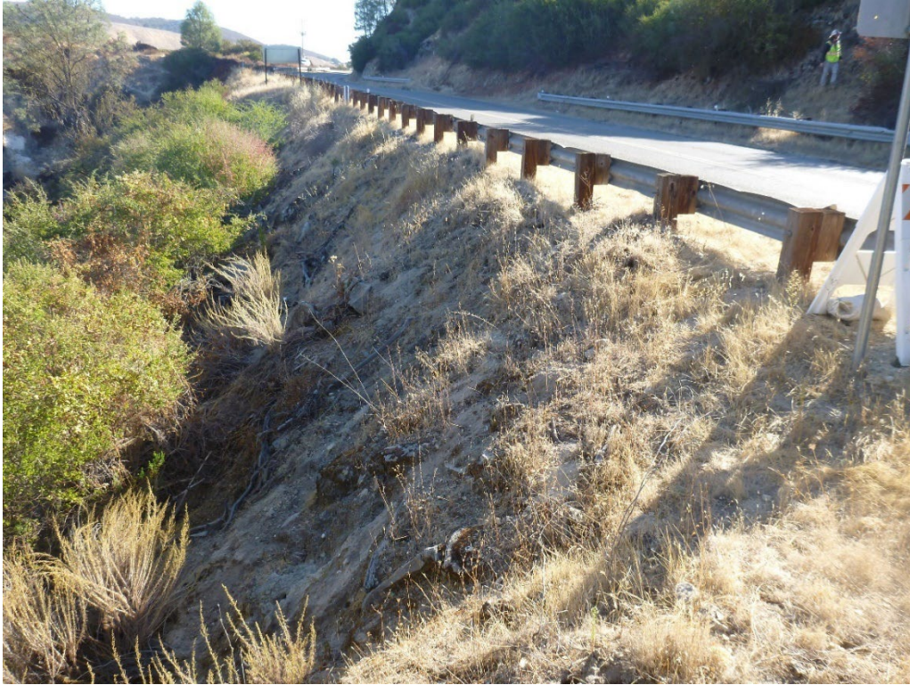
019 Photograph 17 shows the upper flaps (looking east).
