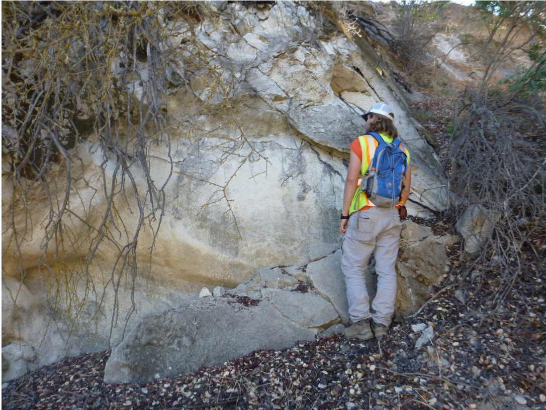
019 Photograph 6. Field site showing roots on failure surface and in fractures in front of the geobags.
