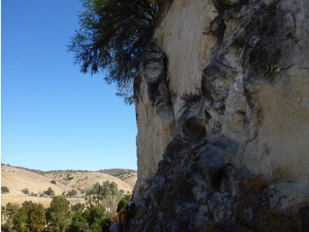
019 Photograph 5. Back cut for access road above Powerhouse. The roots behind the sandstone.
