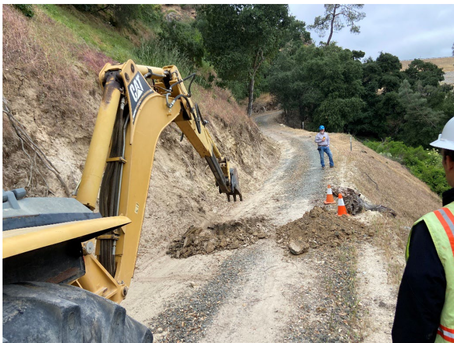
Photo #2: Excavation of TP-1, Looking West
