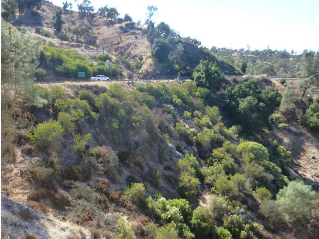
019 Photograph 11. Lake Acireto Dam, showing cuts above road and below
