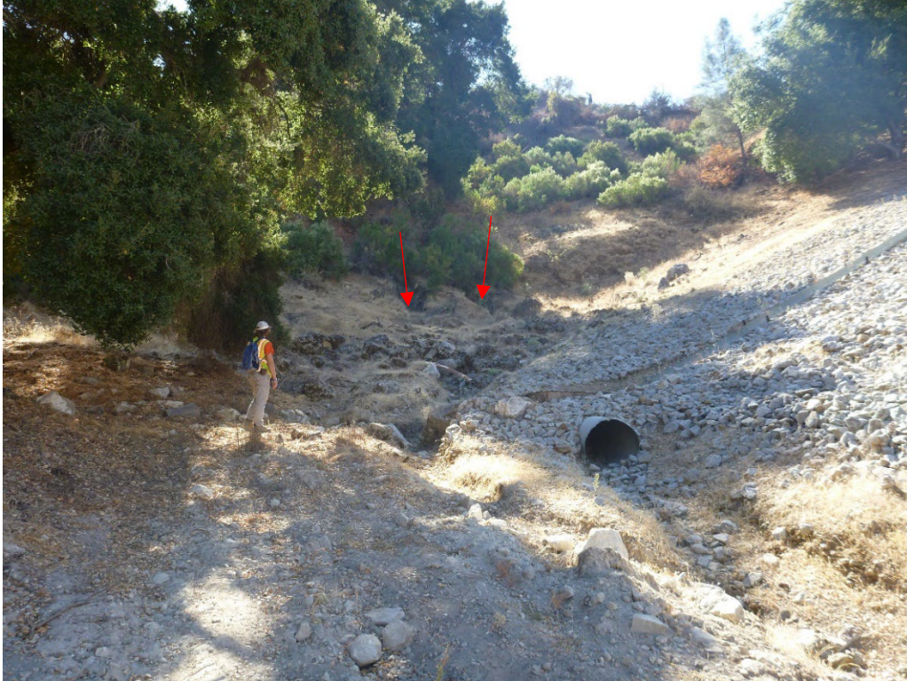
019 Photograph 2019 on the right downstream of the arrow mark the downstream of the gully in Photograph 22.
