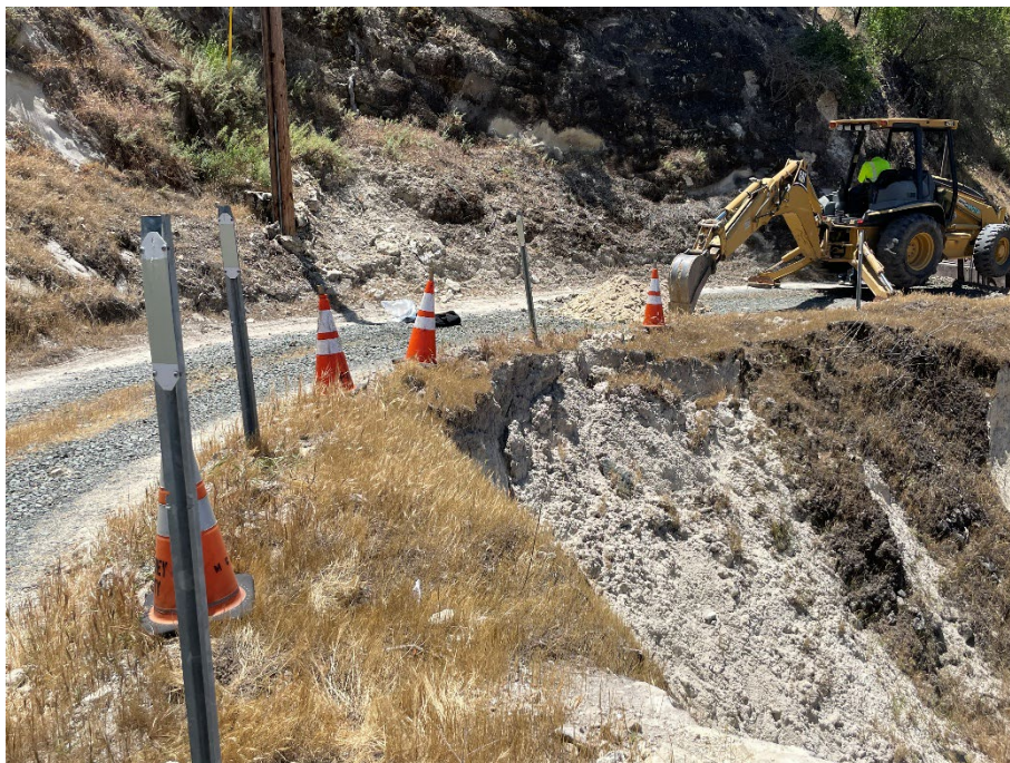
Photo #5: Excavation of TP-3, Looking West
