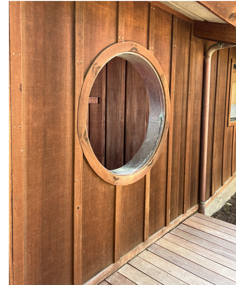
PUMP HOUSE SIDING BOARD AND BATTEN SIDING STAINED TO MATCH EXISTING REDWOOD SIDING AT HOUSE.
