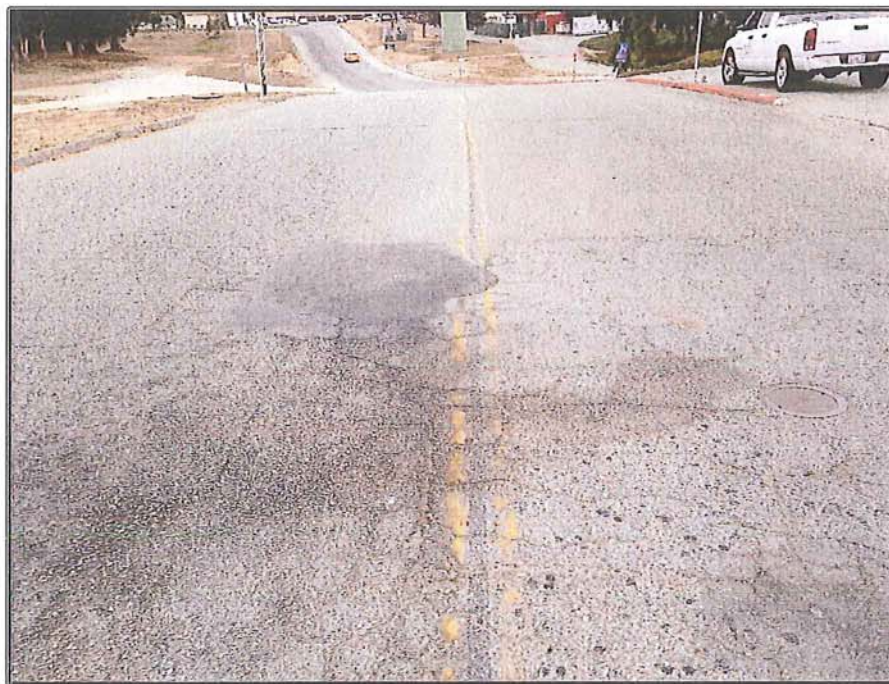
MONTEREY COUNTY JAIL FACILITY PHOTO NO. 6 - NATIVIDAD ROAD TO PERIMETER DRIVE
