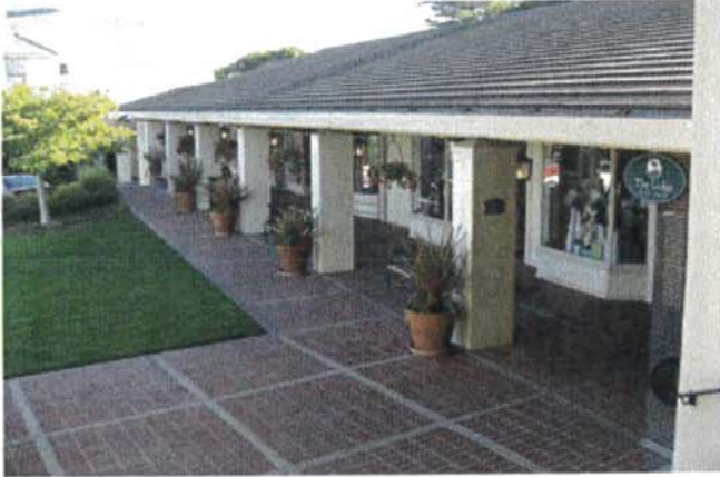
West wing of the Lodge Annex. (Page & Turnbull, November 2012)
