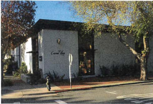
Carmel Plaza, former I. Magnin building. Camera facing southwest. Photo by author.
