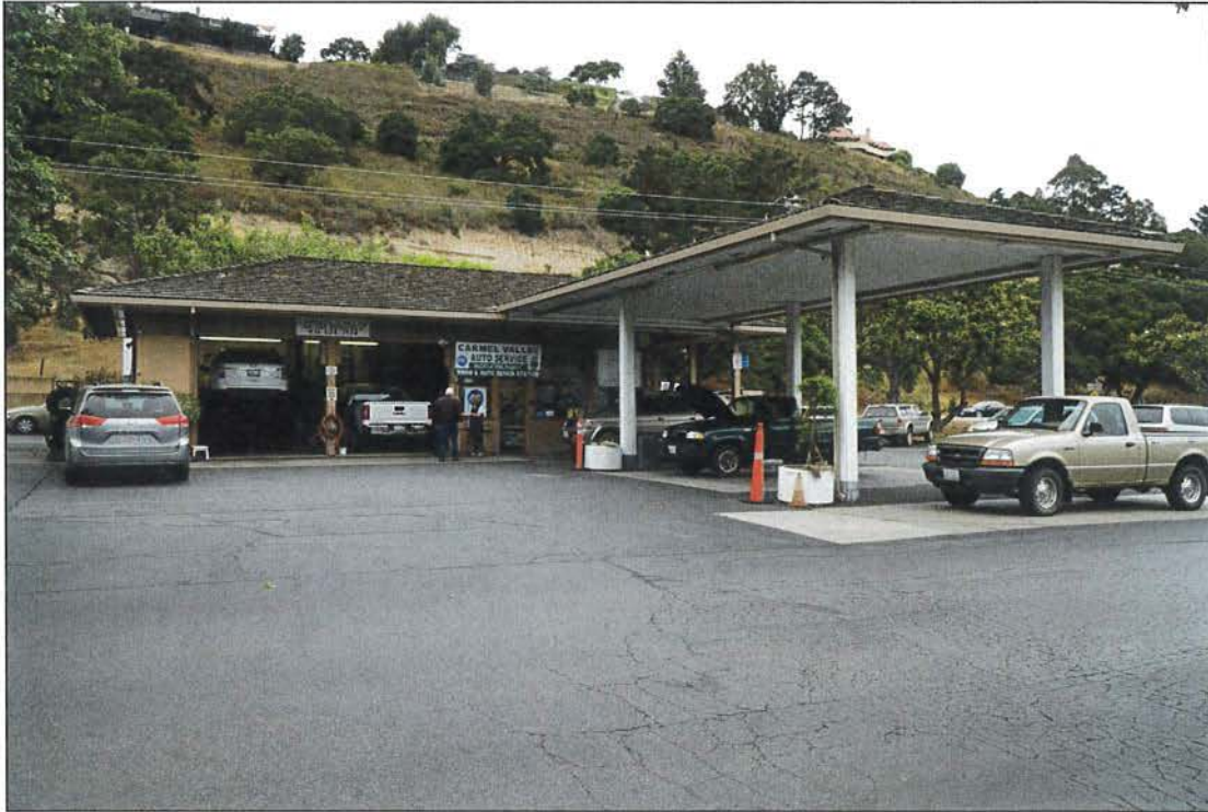
1. Looking northeast at south side of Carmel Valley Auto Service, 19 August 2019. Photograph by Anthony Kirk, Ph.D.
