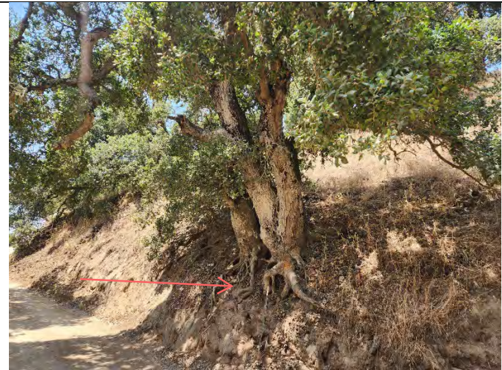
Tree #34; Recommended for removal, soil eroding under tree.
