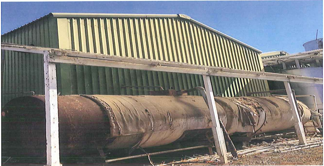
Boilers H – Rear Elevation
