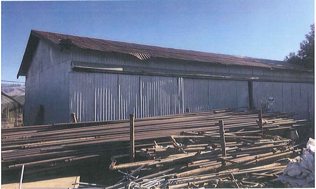
Warehouse C – Rear Elevation
